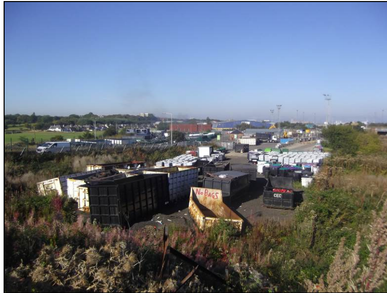
Plate 1: View of proposed development site, facing north-west
