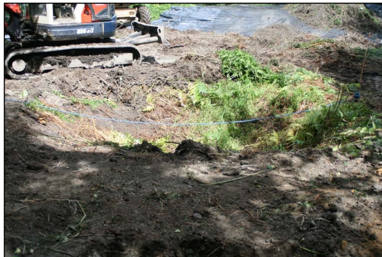
Plate 1: Trench 7 pre excavation
