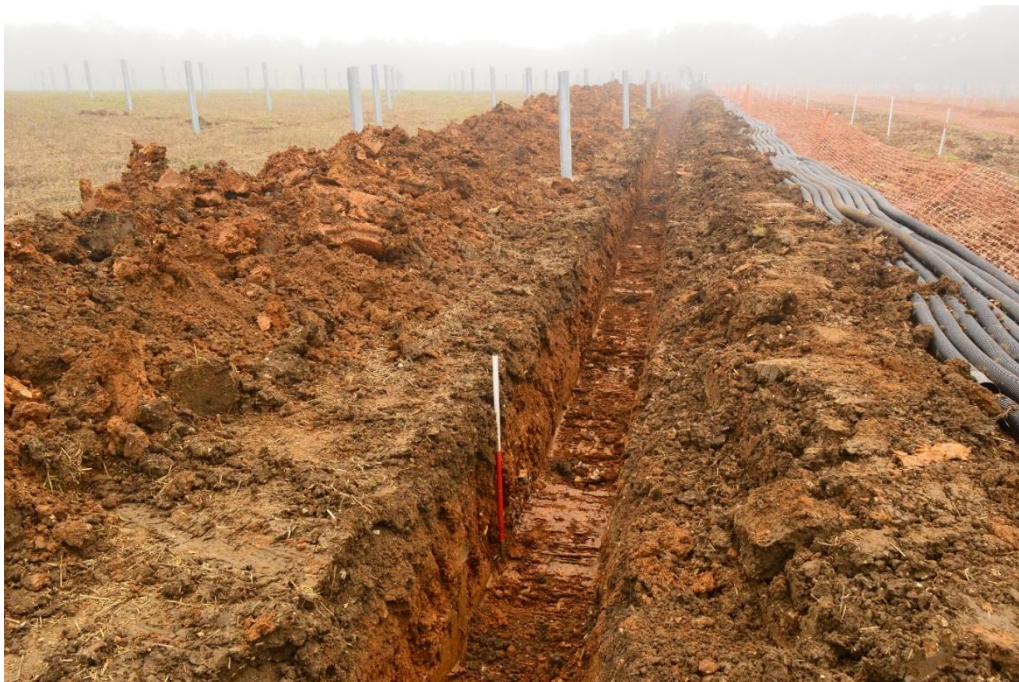
Plate 2; Cable trench in the northern field looking north, scale=1.00m
