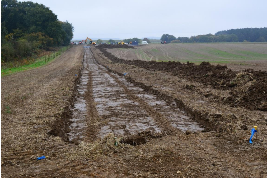
Plate 1; Access road stripped in the northern field, looking north
