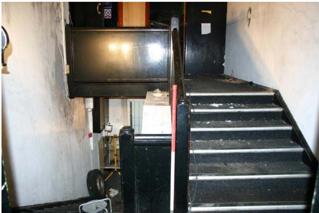
Plate 10: Main staircase, from mezzanine floor
