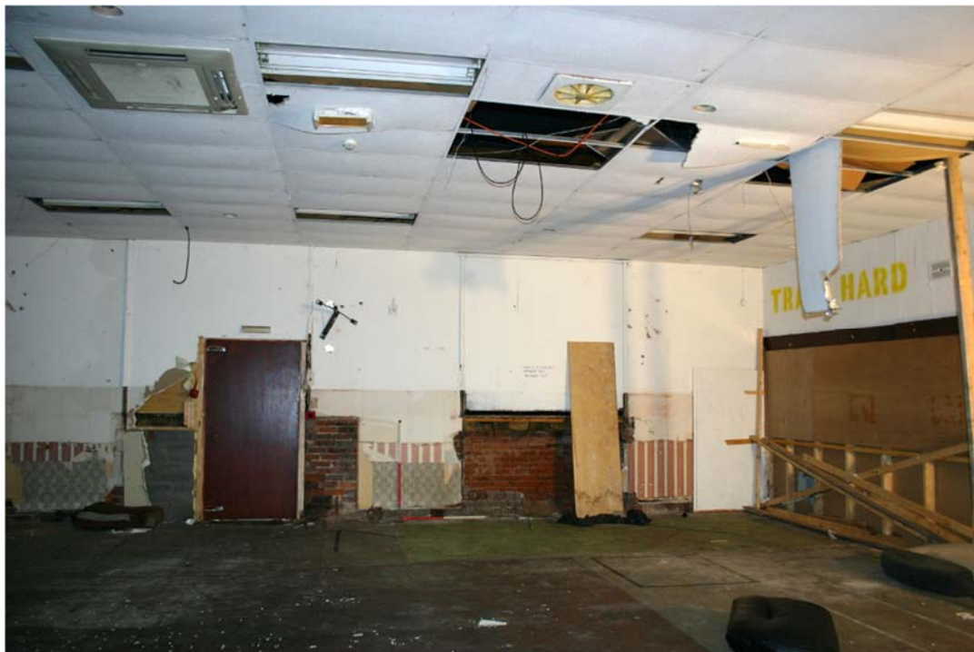
Plate 11: Hall on First Floor, with modern fire escape door and bricked up windows
