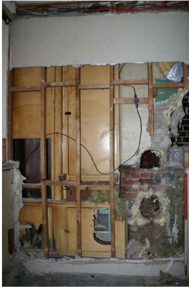
Plate 7: Detail East Elevation of Main Room
