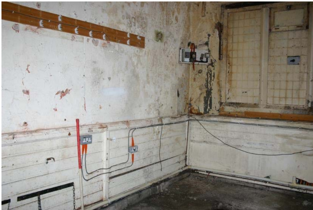
Plate 9: Partitioned off Room on Ground Floor, panelling and original window
