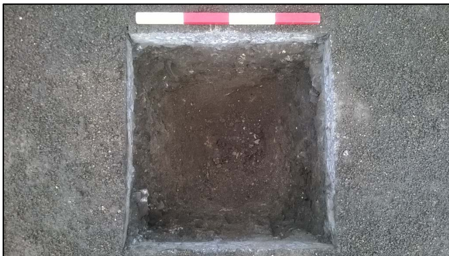
Plate 2; Foundation Pit 2, looking northwest
