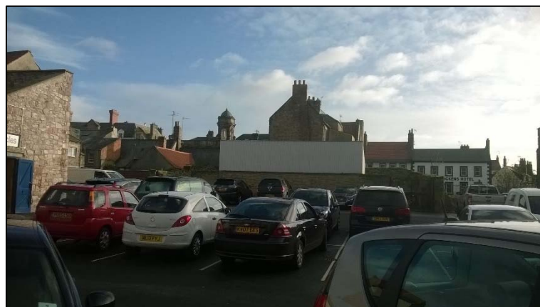
Plate 6: Pumping house to north-west of proposed development site
