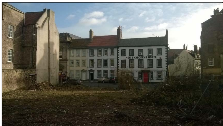
Plate 2: Proposed development site facing north-west
