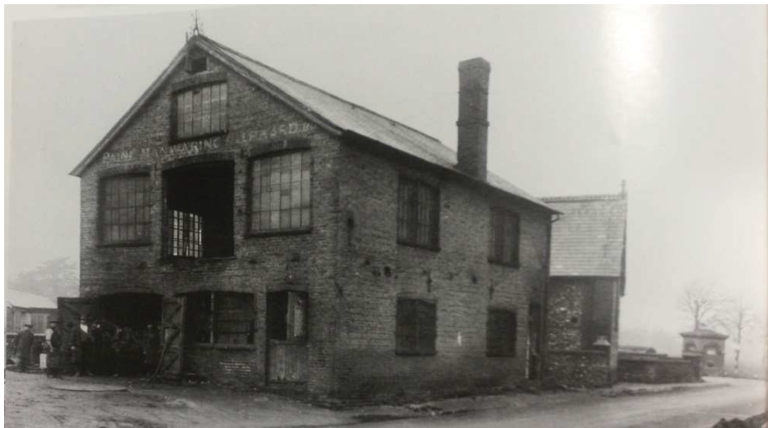
Plate 1: The old smithy, opposite site before demolition, Kerridge & Standing 1983
