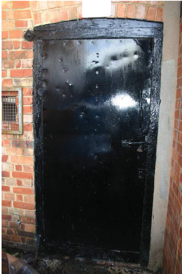
Plate 6: possible original doorway at south elevation of eastern part
