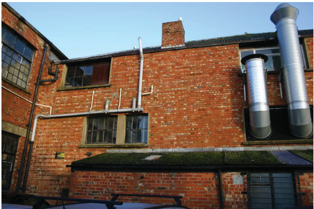
Plate 5: south elevation of eastern part, with outbuilding
