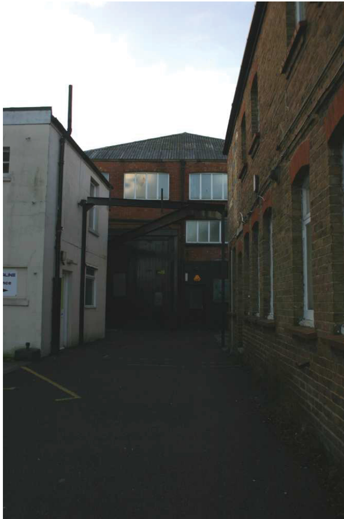
Plate 7: North elevation of building, as seen from Ardsheal Road
