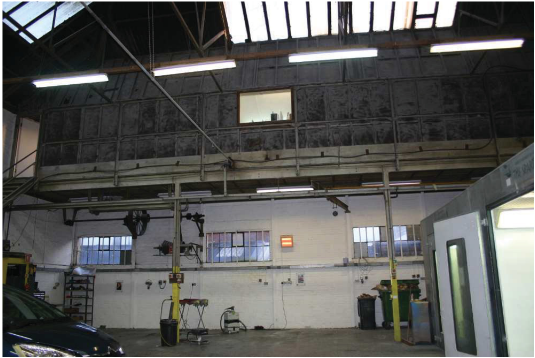
Plate 8: interior of hall, east elevation with galleried floor
