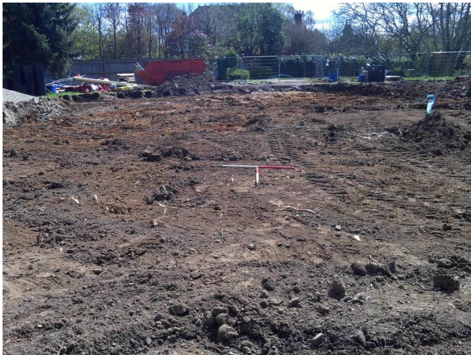
Plate 2; General shot of Trench 2, two 1 metre scales. Looking east.
