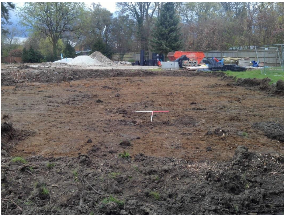
Plate 4; General shot of Trench 3 looking north with two 1 metre scales.
