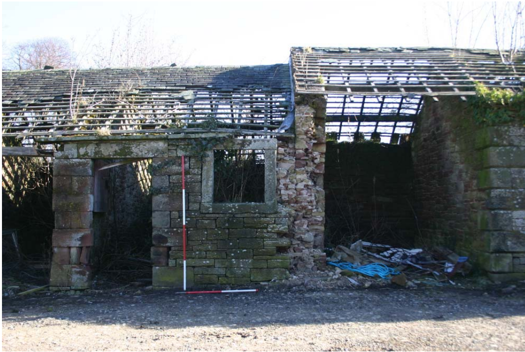
Plate 13: Stable in structure 1 and abutting open space of structure 2
