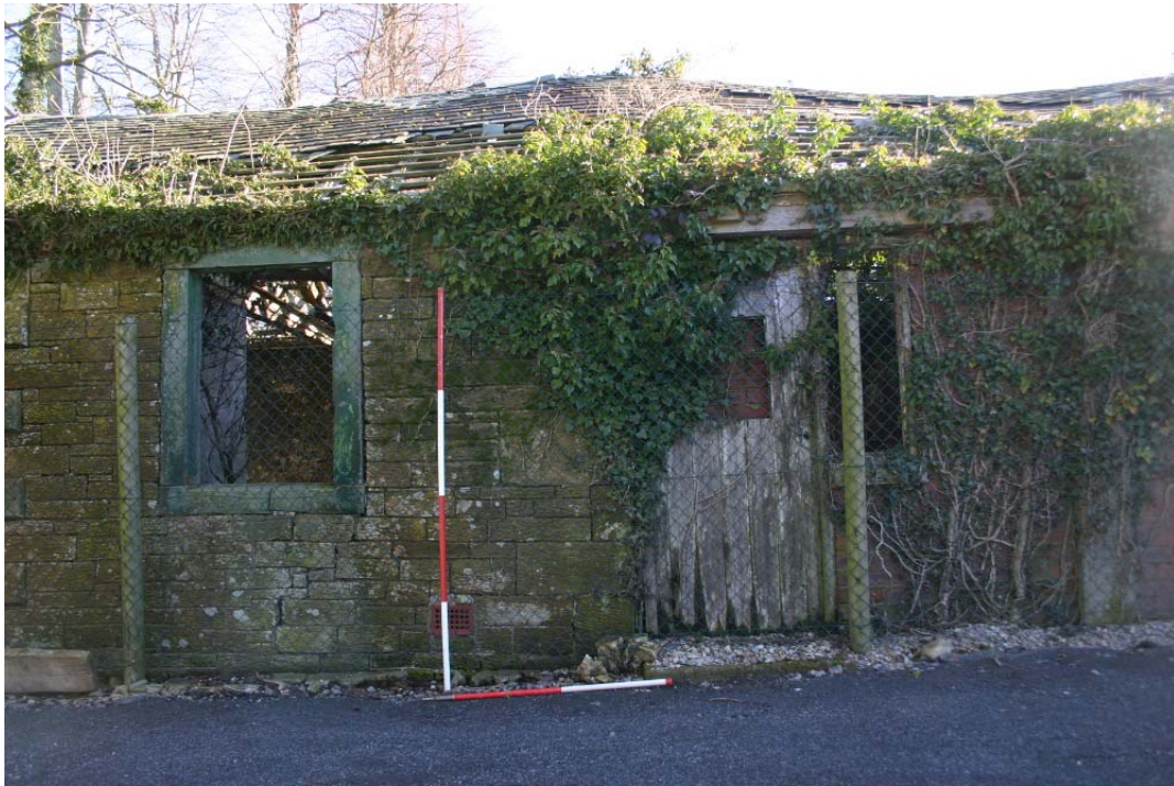
Plate 9: South-west facing elevation, second doorway structure 1
