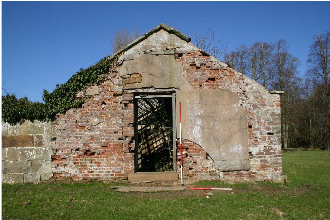
Plate 23: South-east facing elevation, with uncoursed brickwork and sandstone masonry
