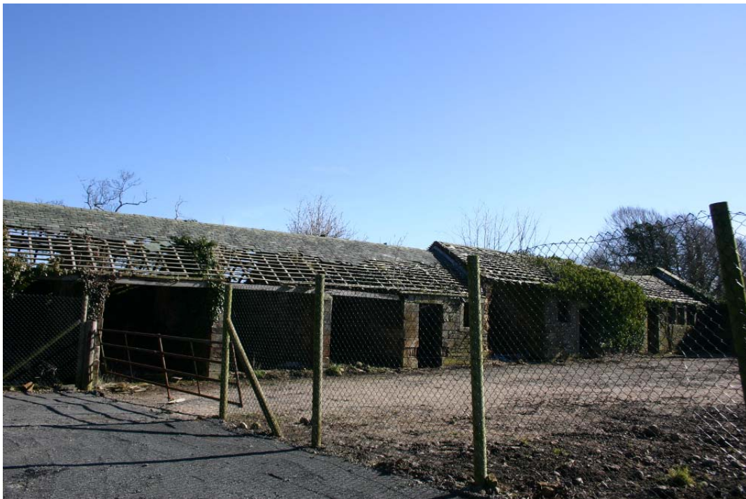
Plate 4: General view South-west elevation 1st and 2nd structure
