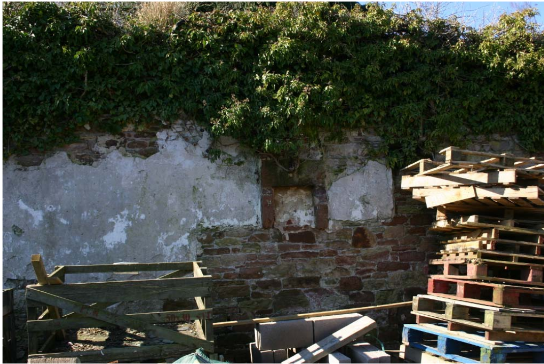
Plate 25: South-west facing elevation of boundary wall with fireplace remains
