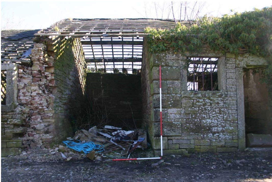
Plate 14: Structure 2, south-west elevation
