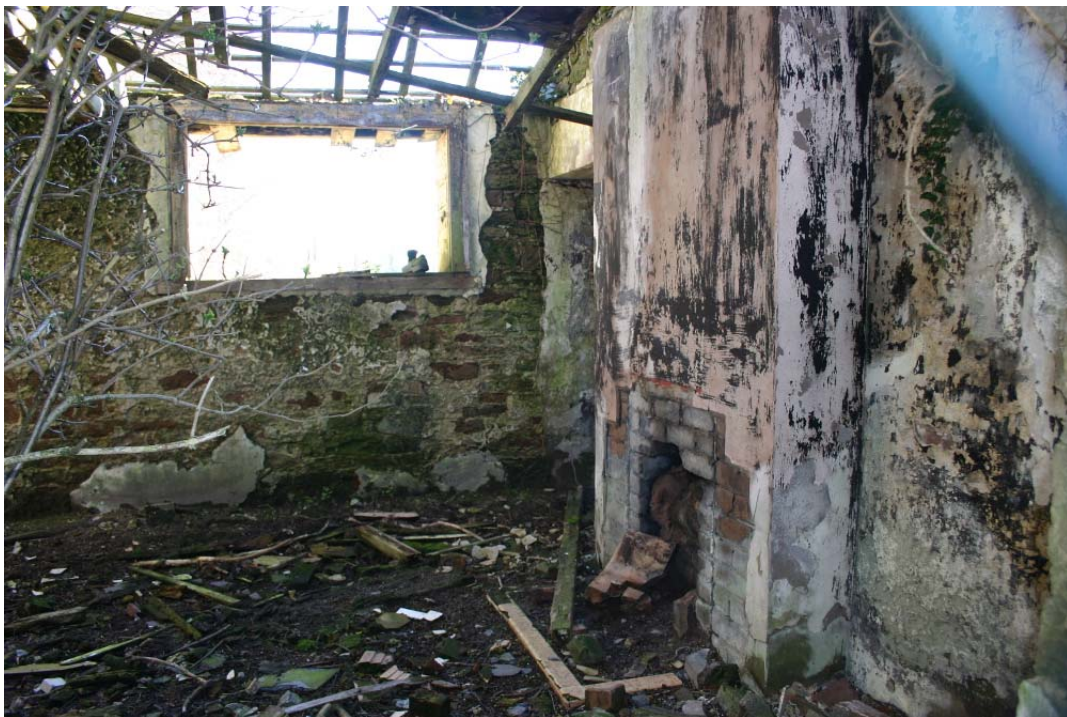
Plate 8: General view 2nd room, structure 1
