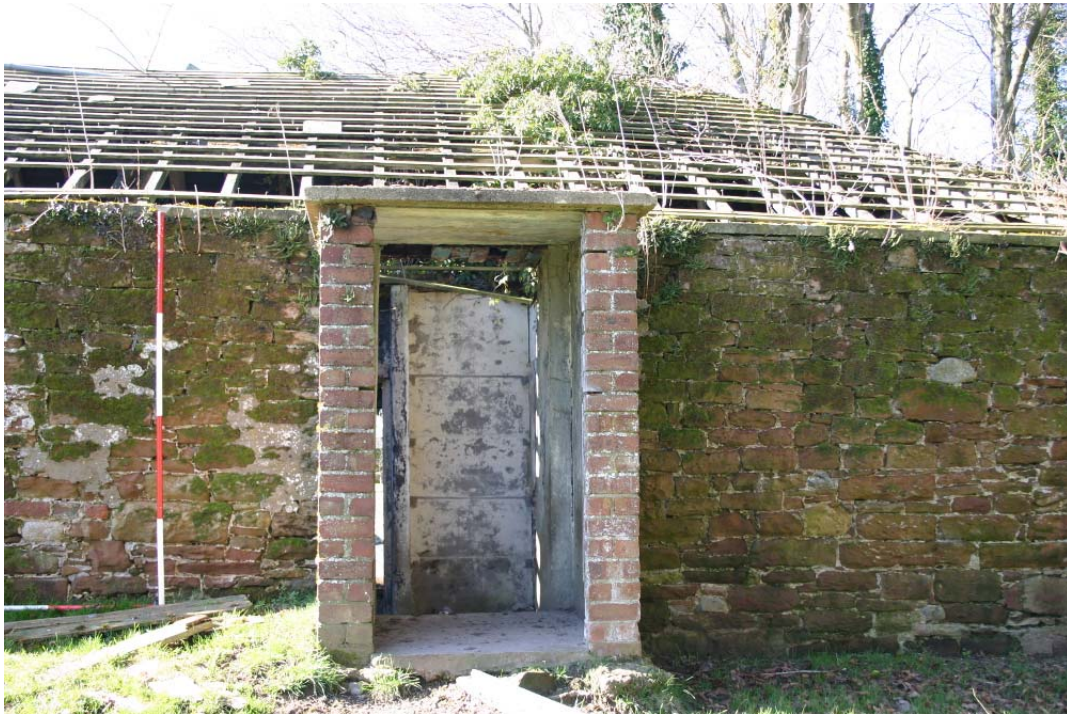
Plate 5: North-east facing elevation of structure 1, modern brick masonry porch
