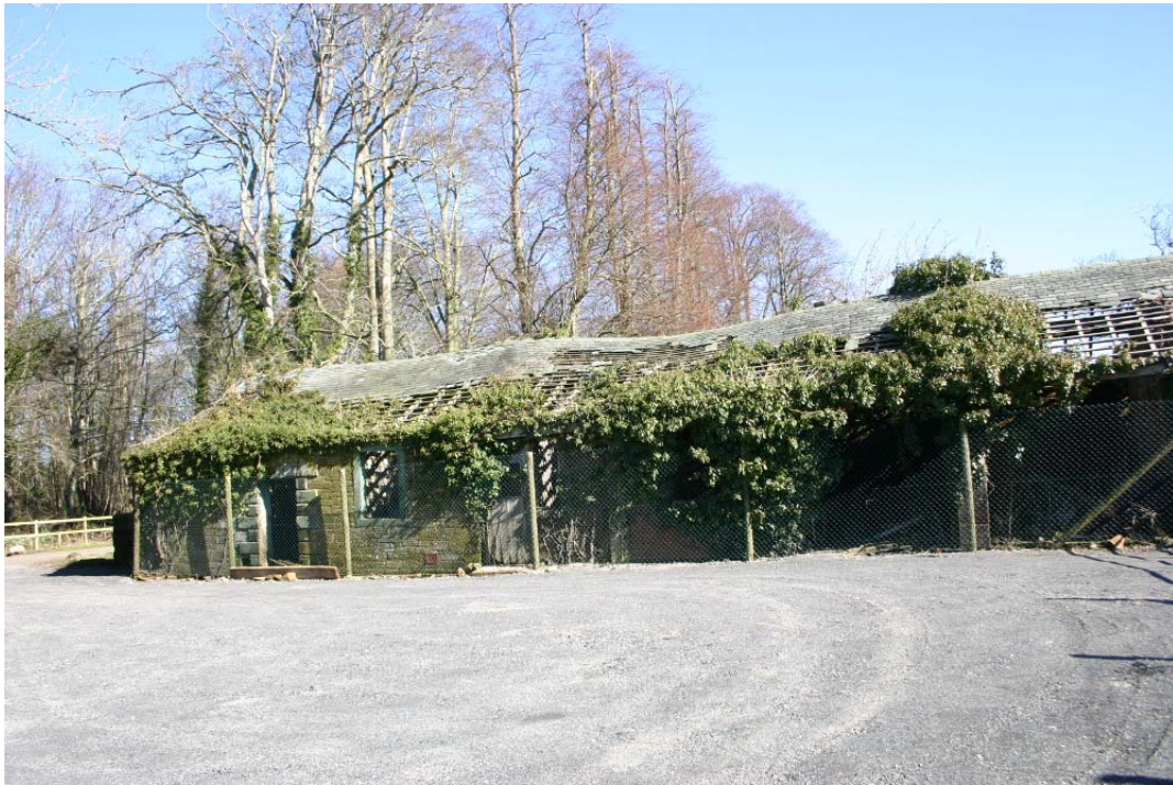
Plate 3: General view of south-west facing elevation, 1st structure
