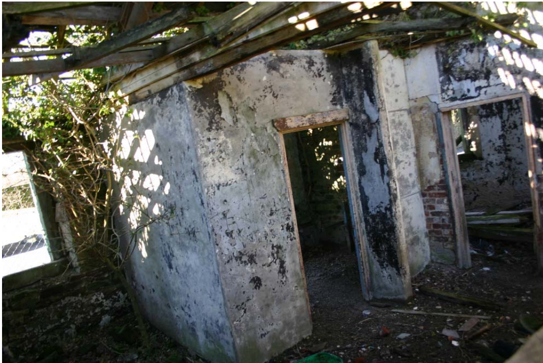
Plate 7: General view, 2nd room, structure 1
