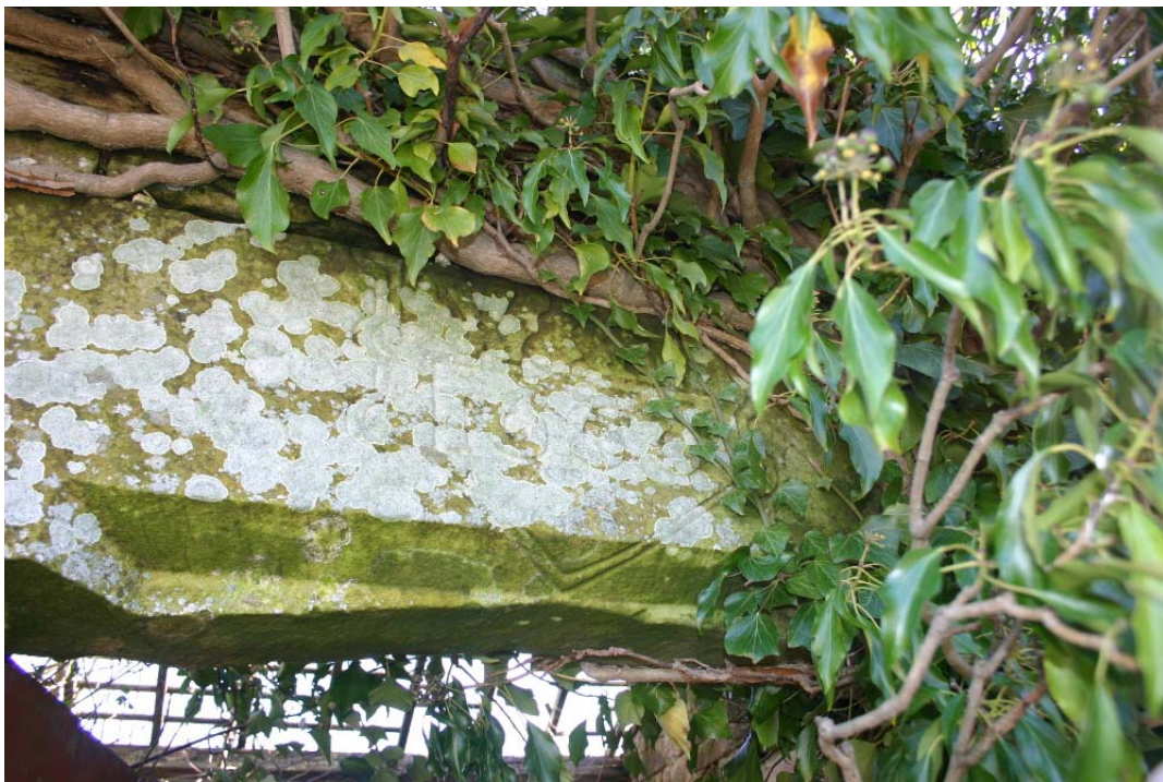
Plate 17: Detail of a reused lintel at south-west elevation, datestone 1660, structure 2
