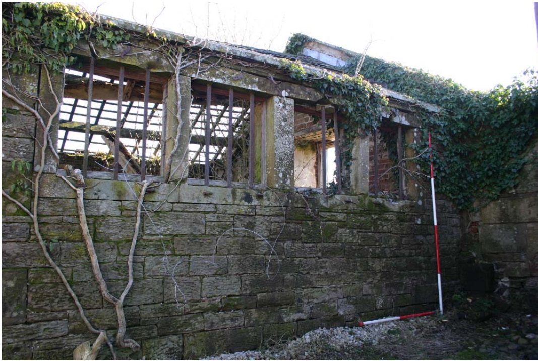
Plate 16: South-west elevation structure 2
