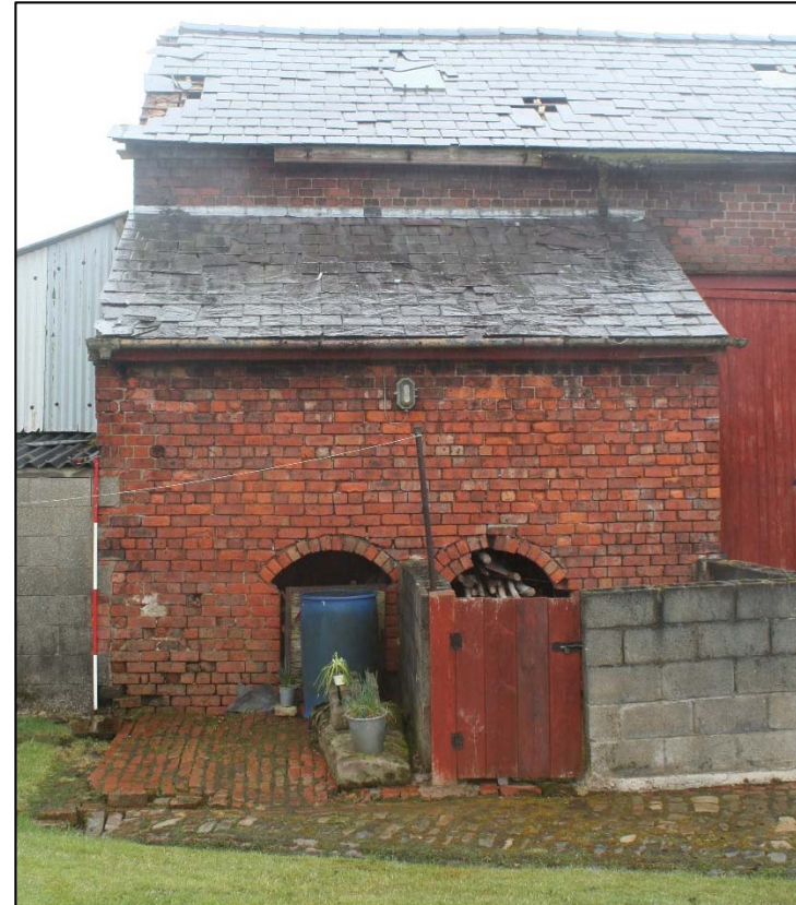
Plate 10: Detail of arched openings in south-west facing extension to Building 2
