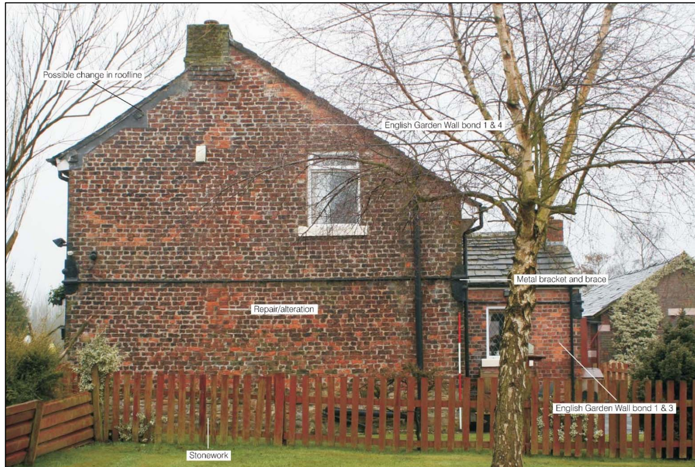
Plate 6: North-east facing elevation of Building 1
