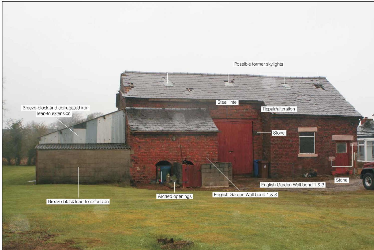
Plate 8: South-east facing elevation of Building 2
