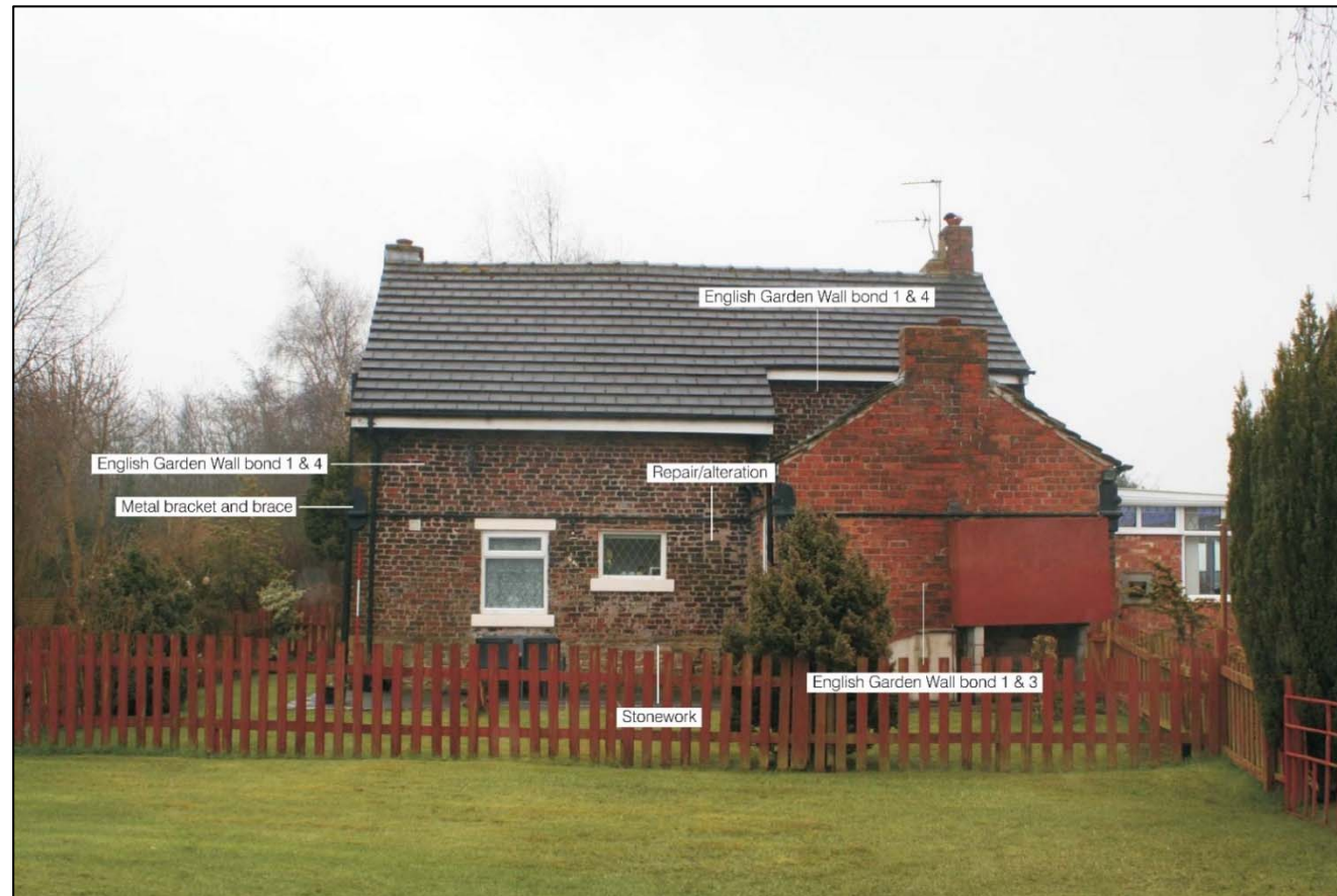
Plate 5: North-west facing elevation of Building 1
