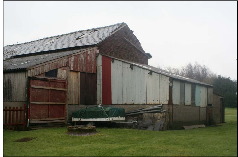
Plate 12: South-west facing elevation of Building 2, from the north
