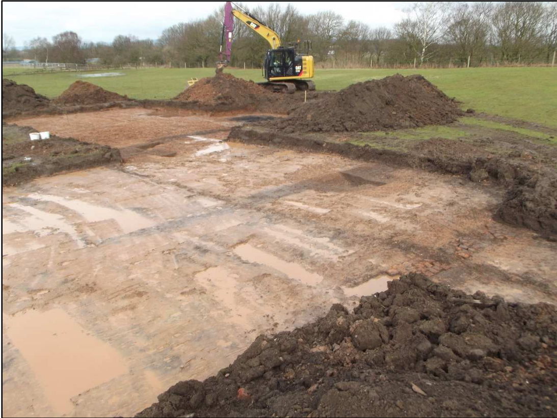
Plate 1; Area 1, looking north
