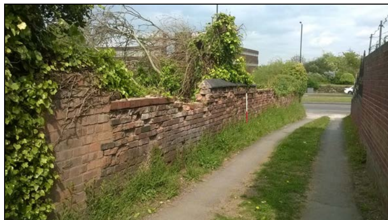
Plate 4: Southern boundary wall of proposed development site, facing north-east
