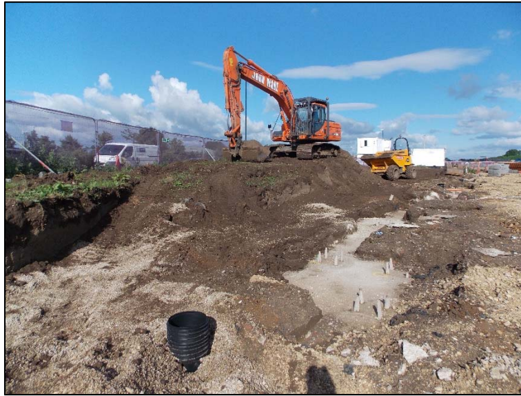
Plate 1: General view of bund removal, facing west
