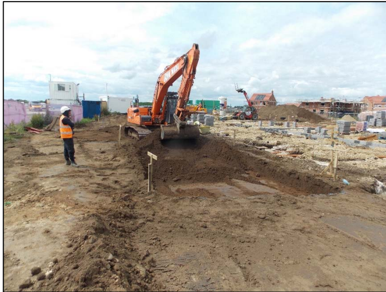
Plate 3: Excavating to final depth, facing west-north-west
