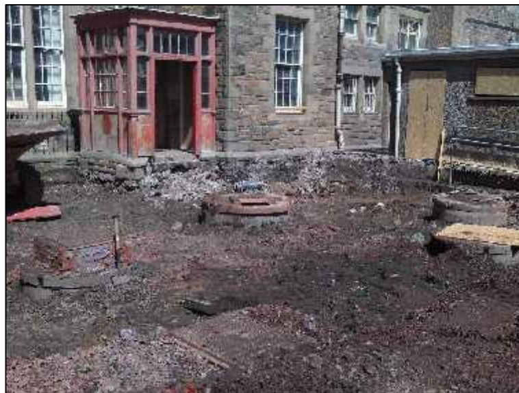
Plate 2: Services encountered during groundworks, facing north
