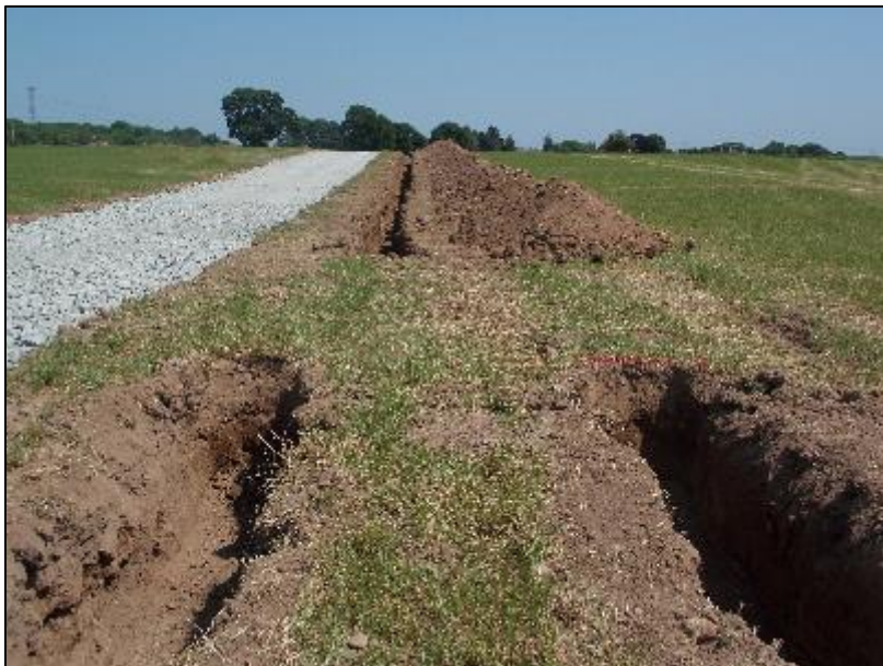
Plate 1; Trenches 3, 4 and 6 looking west
