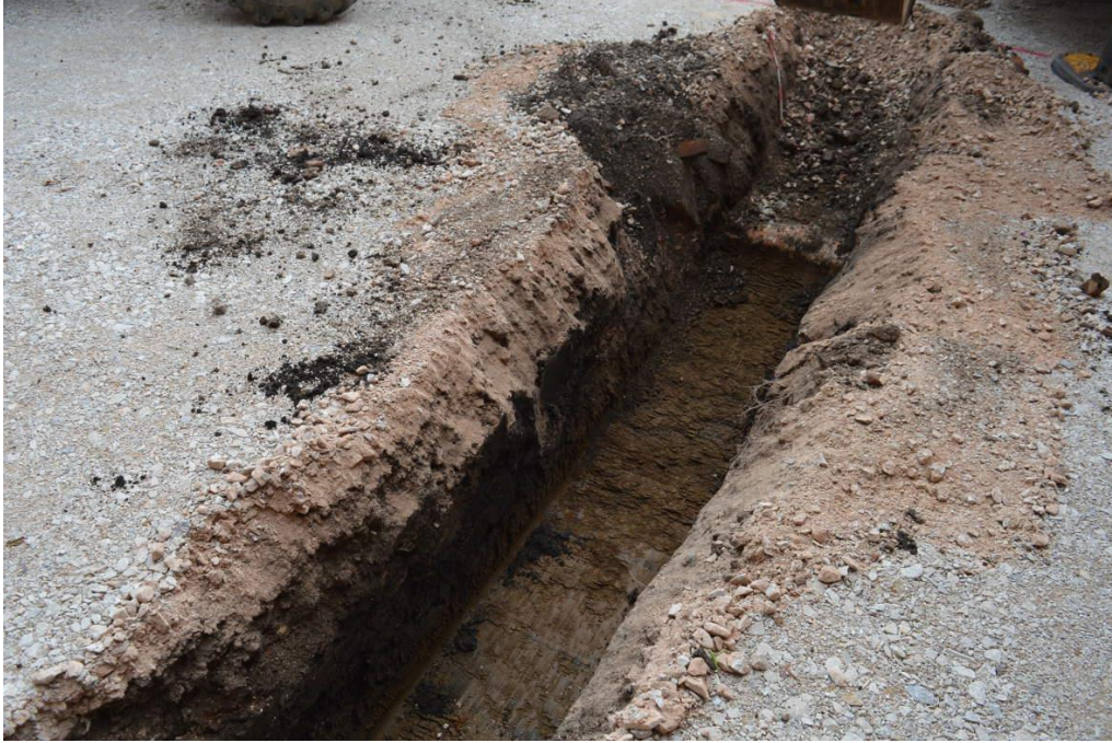
Plate 1; Clay at base of south side of foundation trench (facing north east)
