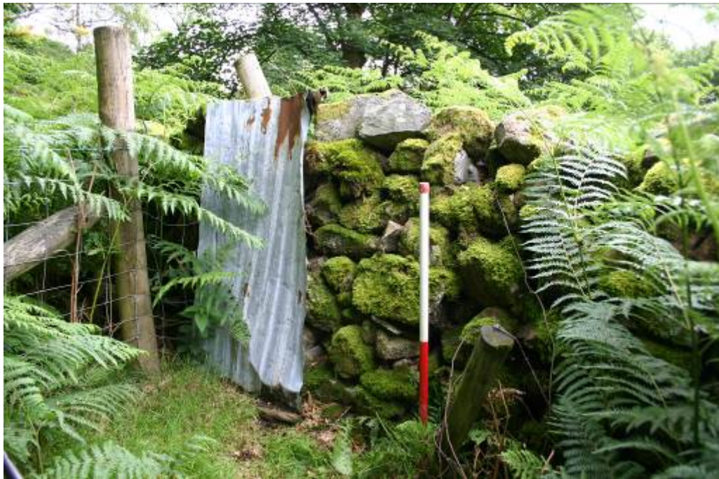
Plate 1: Remains of building, north-north-west facing elevation
