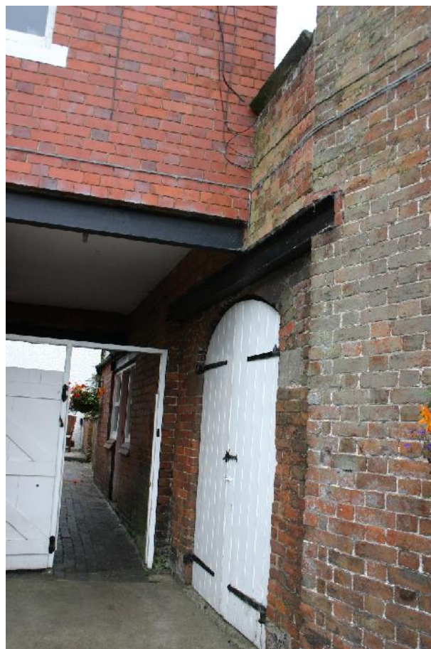
Plate 12: Extension shed partially to be demolished
