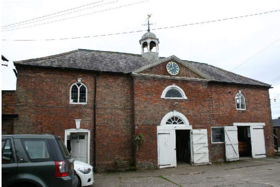
Plate 1: North-east facing elevation with clock face
