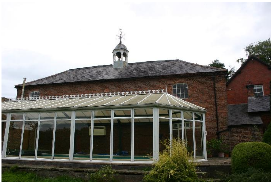
Plate 4: South-west facing elevation, with modern pool extension
