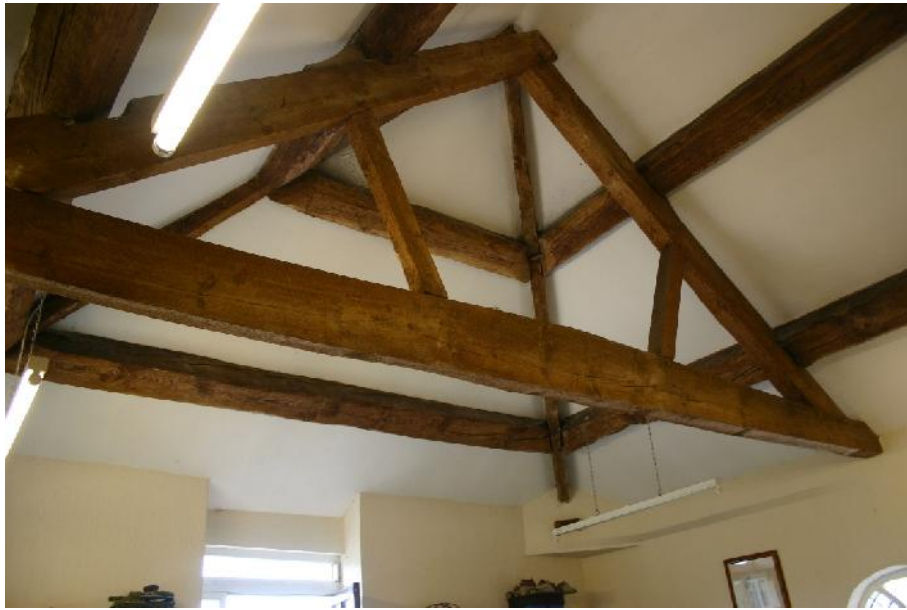
Plate 9: exposed roof timbers in westernmost first floor room
