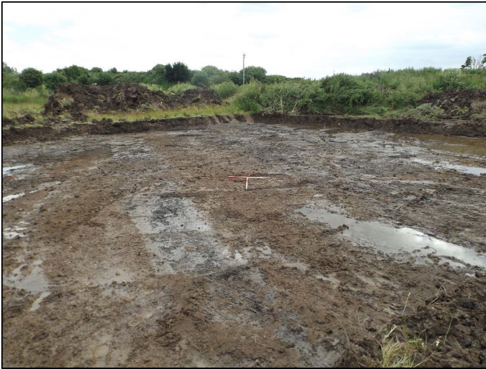
Plate 1: Trench 1 looking south east.
