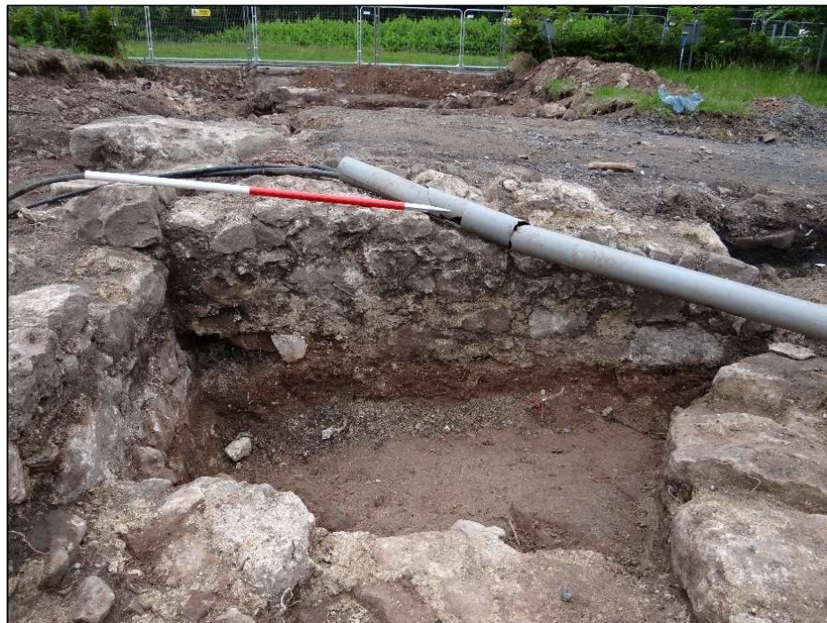
Plate 10; South facing elevation of wall {122}
