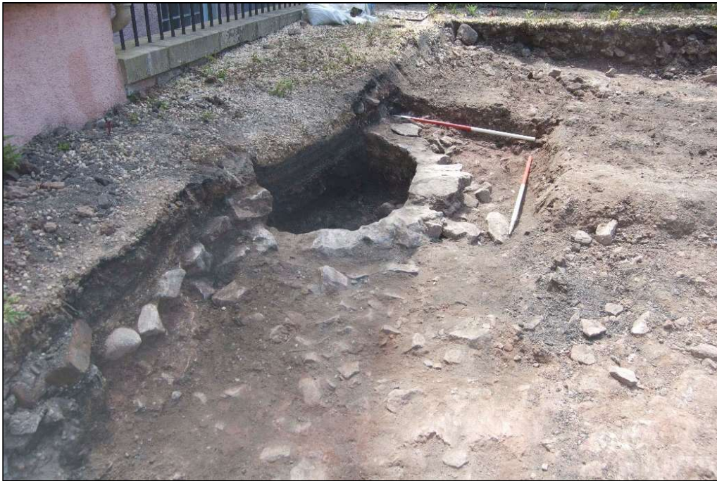
Plate 11; View southeast of well {113}
