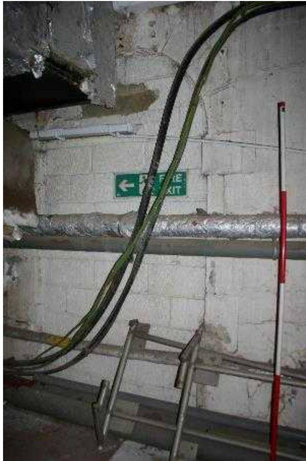
Plate 16: Lift Tower, TF-4, blocked archway at west elevation
