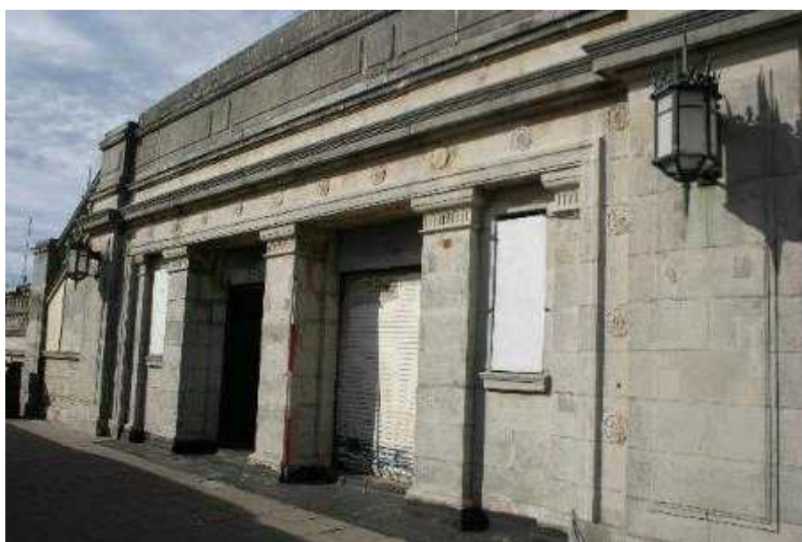
Plate 36: South facing elevation of southern balustrade, closed entrance to aquarium
