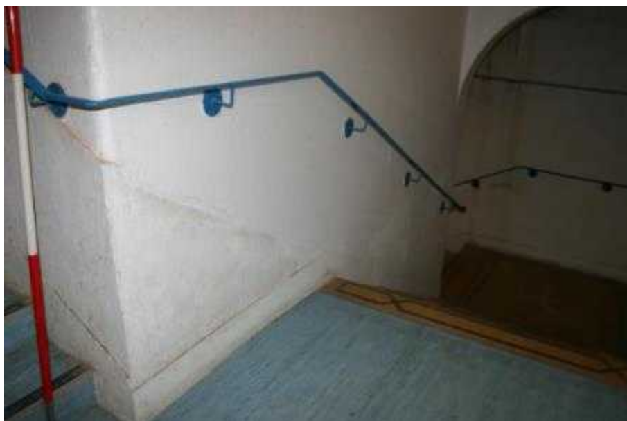
Plate 7: Lift Tower, third storey, alteration at central hoistway
