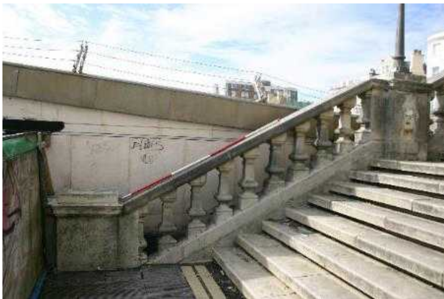
Plate 30: Balustrade/handrail at western staircase of tower
