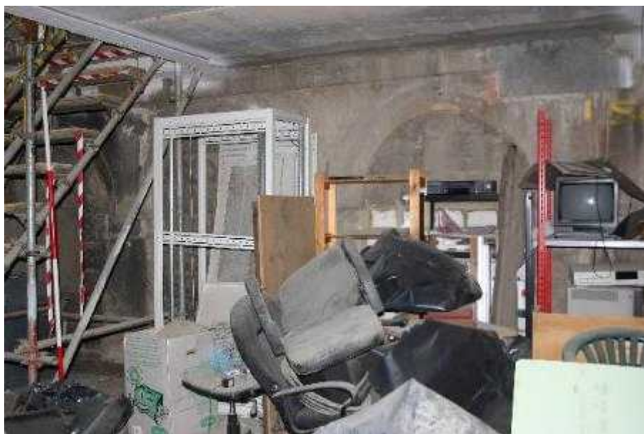
Plate 19: Unit 6 Basement, blocked archways
