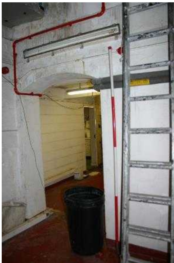
Plate 14: Lift Tower, TF-2, archway to TF-3
