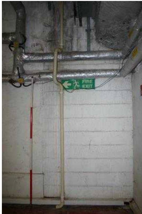
Plate 13: Lift Tower, TF-2, blocked archway east elevation
