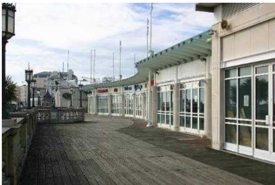
Plate 32: southern balustrade and modern structures, general view
