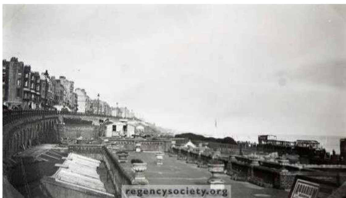
Plate 40: 1927 Terrace before demolition and rebuilt, http://www.regencysociety-jamesgray.com/
