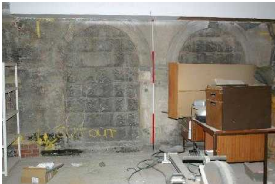
Plate 18: Unit 6 Basement, blocked archways
