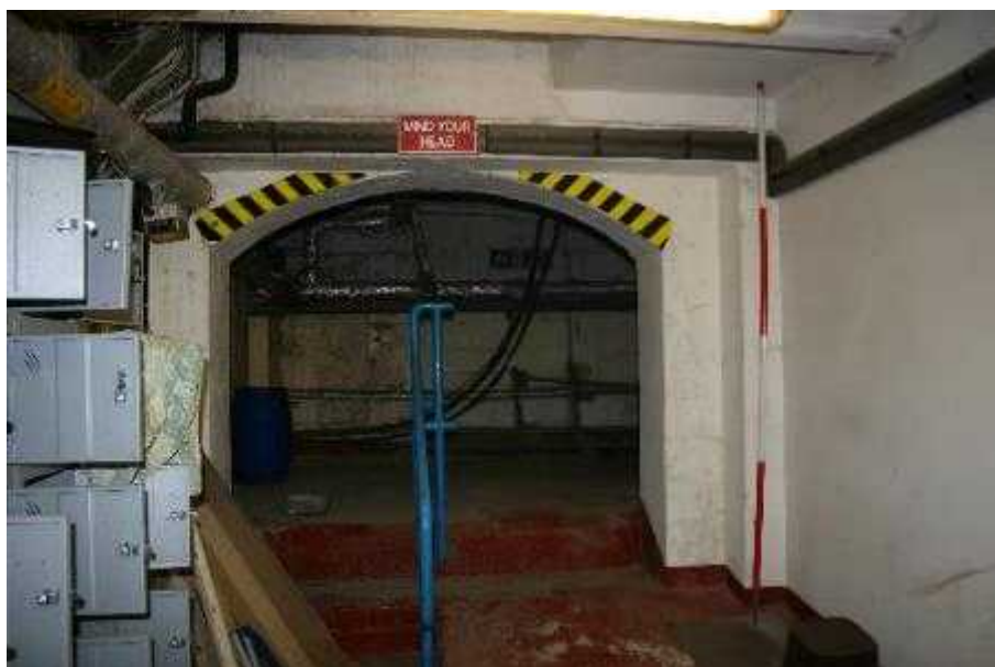
Plate 15: Lift Tower, TF-3, archway to TF-4
