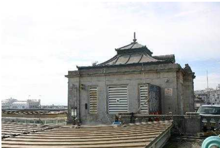
Plate 5: Lift Tower, East facing elevation
