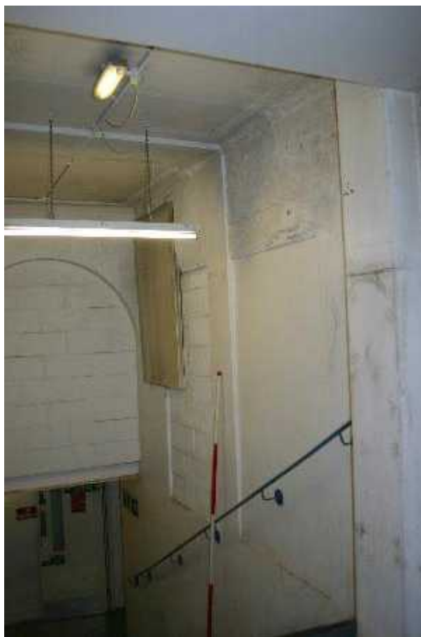
Plate 6: Lift Tower, second storey, blocked opening and round arch
