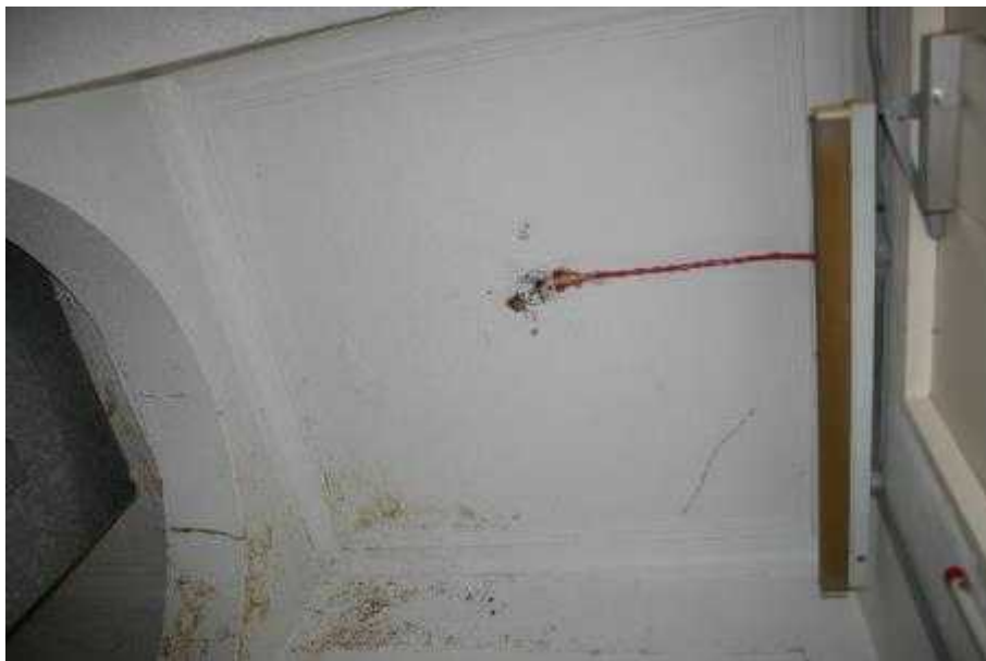
Plate 9: Lift Tower, half-landing between third and fourth storey, coving
