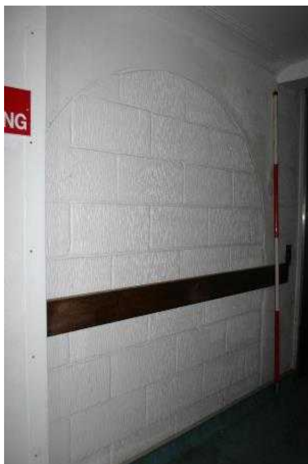
Plate 22: Corridor Unit 5 and 6, blocked arch at south elevation
