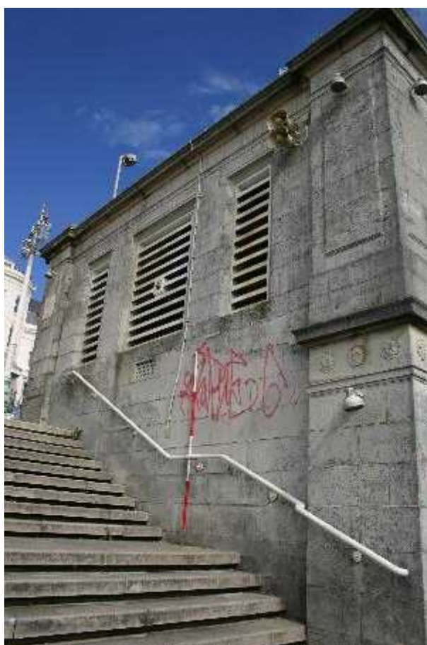
Plate 3: Lift Tower, West facing elevation
