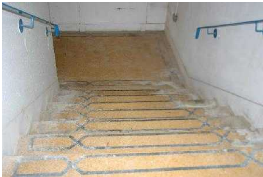
Plate 10: Lift Tower, staircase to fourth storey
