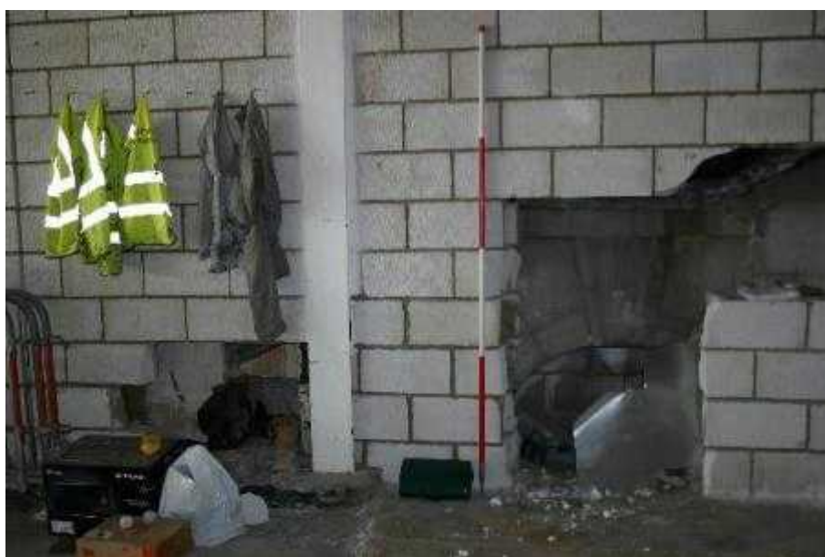
Plate 20: Unit 6, remains of arch at west elevation
