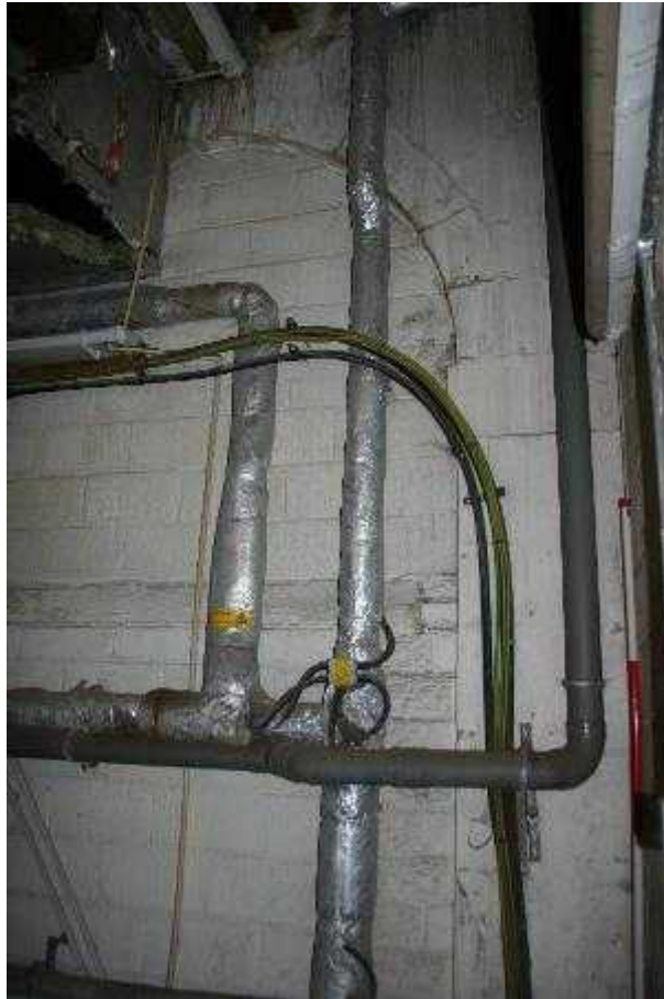
Plate 17: Lift Tower, TF-4, blocked archway at west elevation
