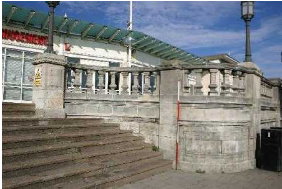
Plate 37: south facing elevation of southern balustrade, main staircase
