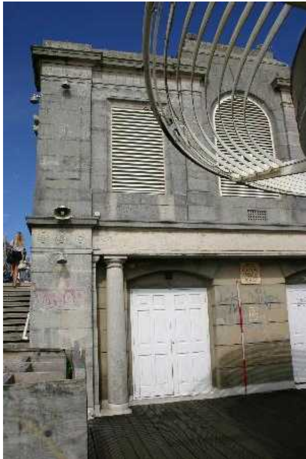
Plate 1: Lift Tower, South facing elevation
