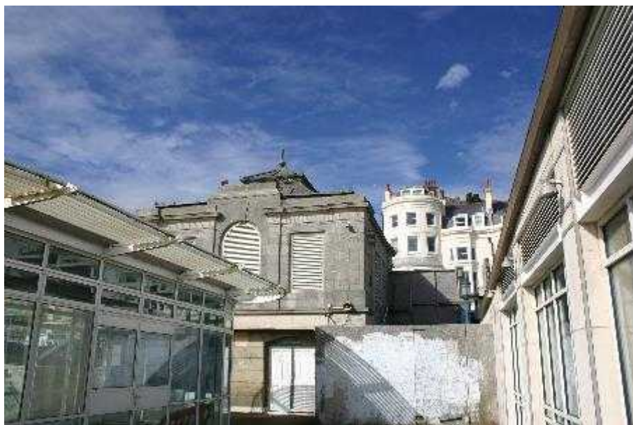
Plate 2: Lift Tower, South facing elevation
