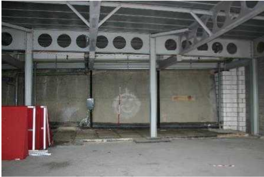
Plate 25: Unit 7, outlines and drainage channel, angled north elevation
