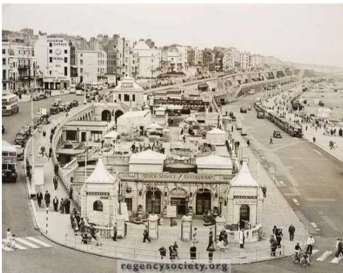
Plate 45: 1952, several small structure have been built on top of terrace, http://www.regencysociety-jamesgray.com/
