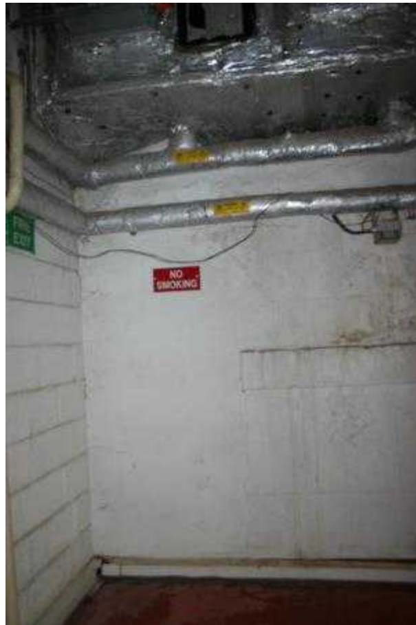
Plate 12: Lift Tower, TF-2 south elevation blocked archway
