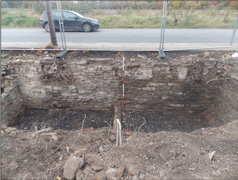
Plate 3; View north-northwest of Cellars 2a and 2b
