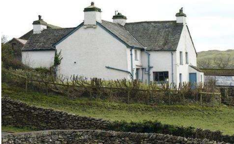
Plate 15: east view of the farmhouse, asset 7, http://www.geog.port.ac.uk/webmap/thelakes/html/lgaz/lk20636.htm
