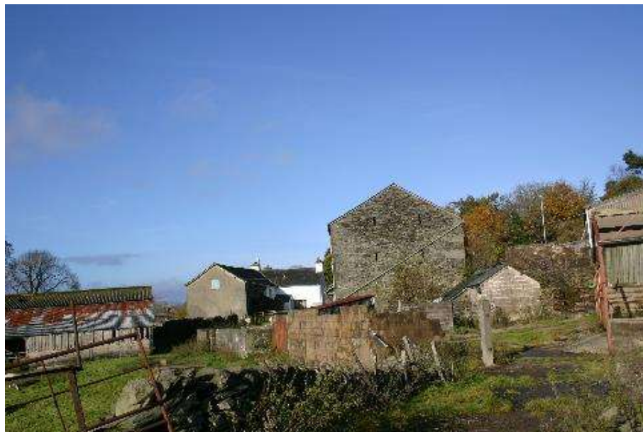
Plate 21: General view of the farmstead
