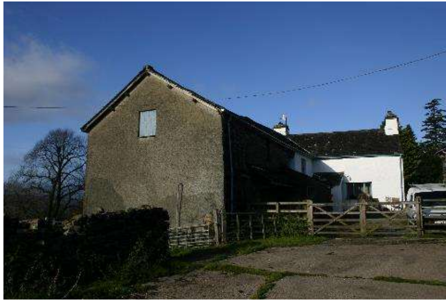
Plate 16: North facing view of the farmhouse, asset 7
