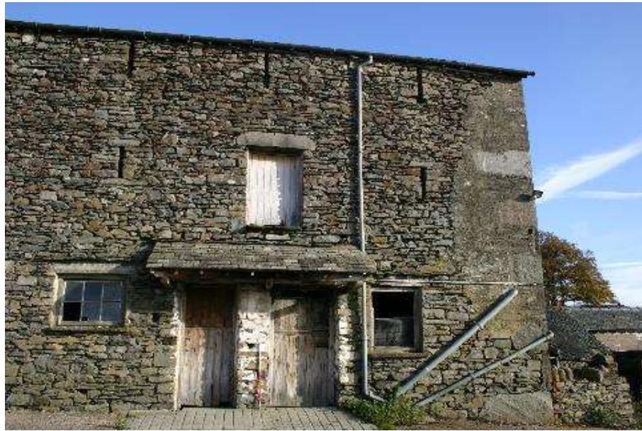
Plate 18: General view of the three storey barn, with modern alterations visible
