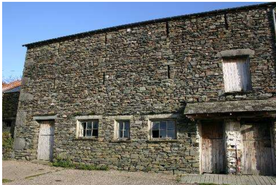
Plate 17: General view of the three storey barn
