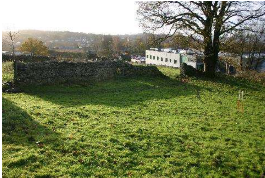
Plate 24: Boundary wall, several phases of construction visible, possible site of previous outbuildings
