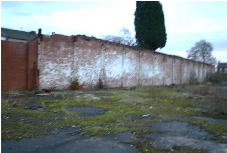
Plate 6: Brick wall at the eastern extend of the site
