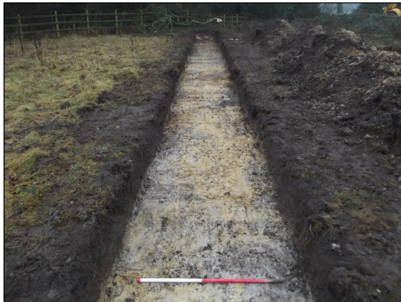
Plate 8 – Trench 3 overview, looking west south - west, 1 x 1m scale
