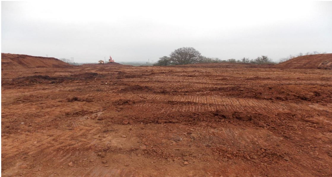
Plate 1; Pre-ex shot of site. Looking northeast. No scale
