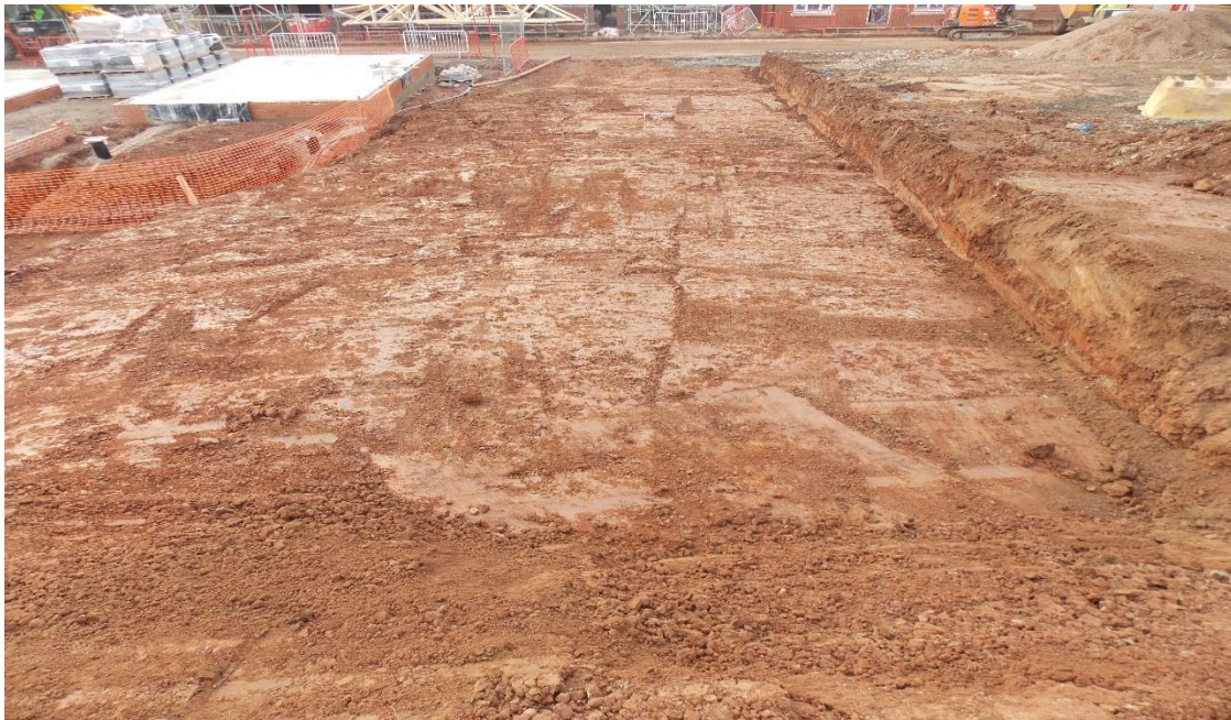
Plate 2; New access road. Looking northwest. 2x1m scales
