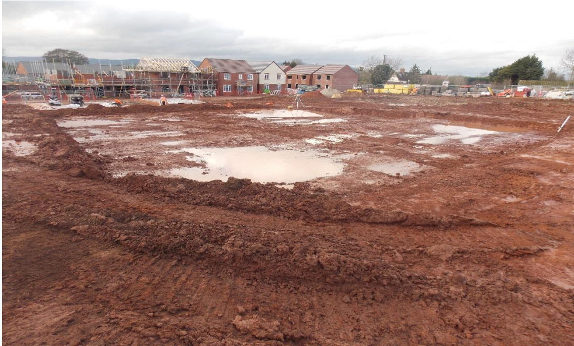
Plate 5; Excavated site showing natural substrate (2002). Looking west. 2x1m scales
