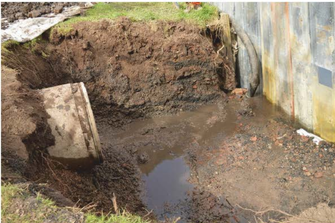
Plate 4; East facing section of excavations. Facing west.
