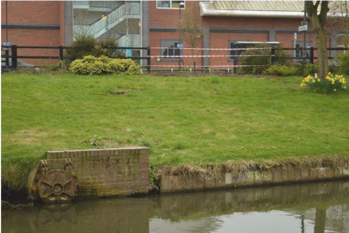
Plate 1; Pre-excavation image of headwall. Facing southwest.
