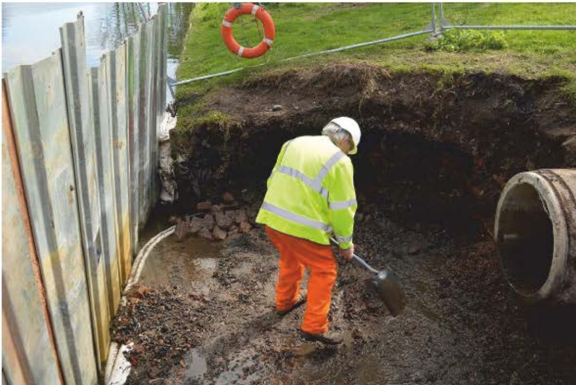
Plate 5; Working shot showing west facing section of excavations. Facing east.
