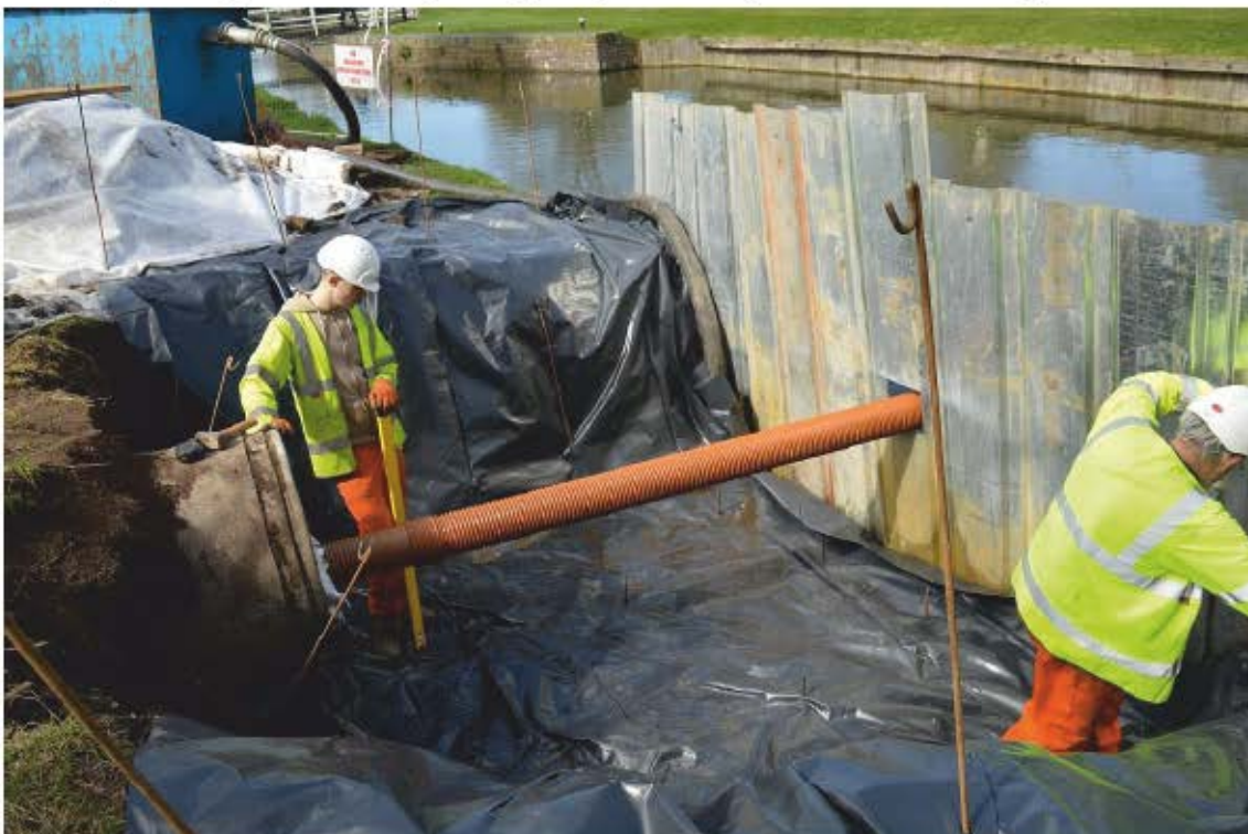
Plate 6; Working shot of plastic membrane insertion over geotextile. Facing west.
