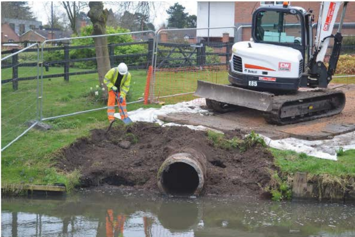
Plate 3; Working shot during initial intrusive works. Facing south.
