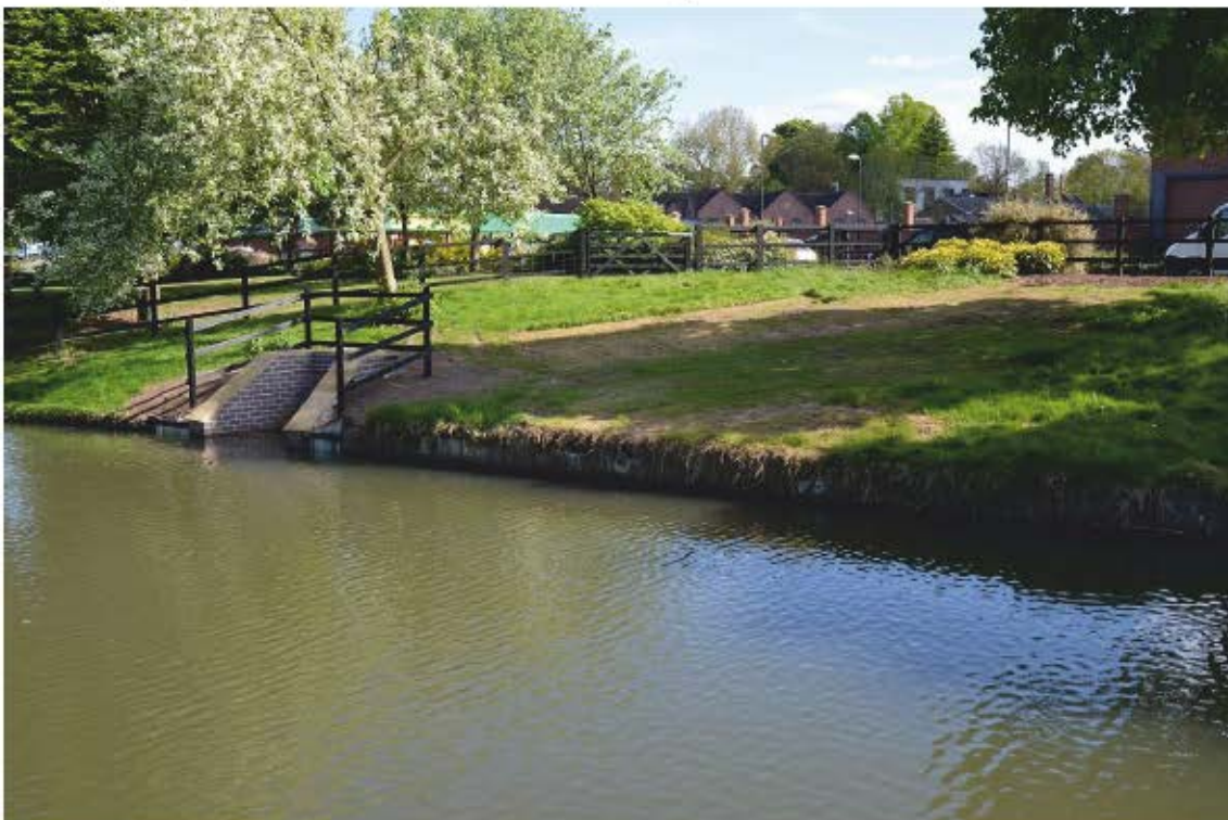
Plate 8; General view of completed storm water headwall. Facing southwest.
