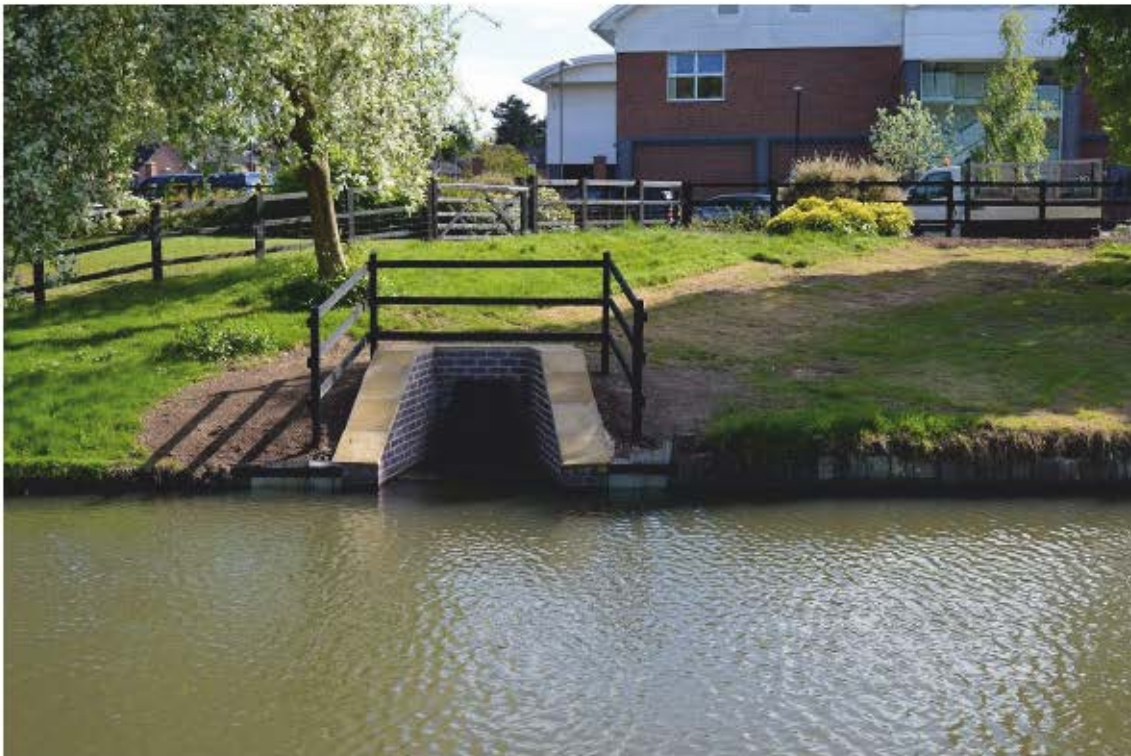
Plate 7; Completed storm water headwall. Facing south.
