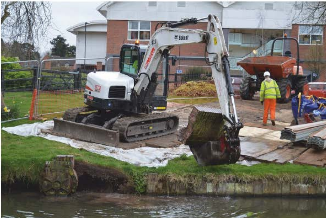
Plate 2; Demolition of headwall. Facing south.
