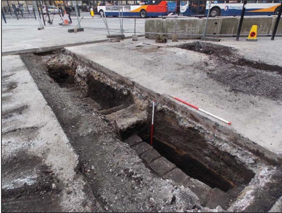
Plate 1; Trench 1, looking southwest (1m scale)
