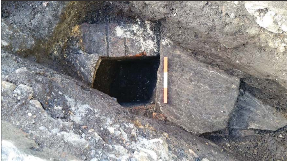
Plate 13; Culvert {309}, looking southwest (30cm scale)
