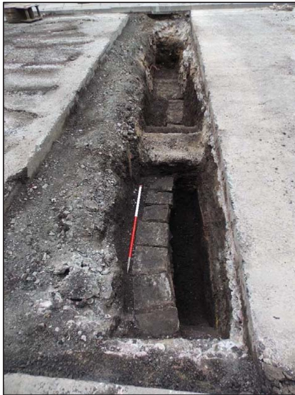
Plate 4; Culvert {108}, looking south-southwest (1m scale)
