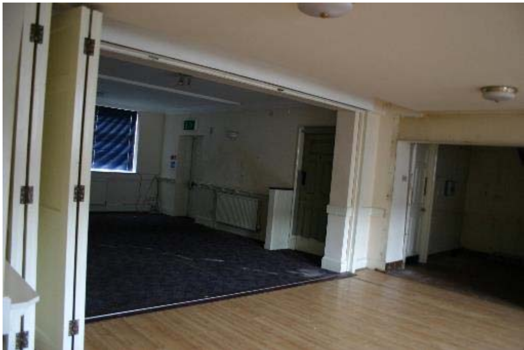
Plate 6: No 16, basement floor, greatly altered for Liberal Club use
