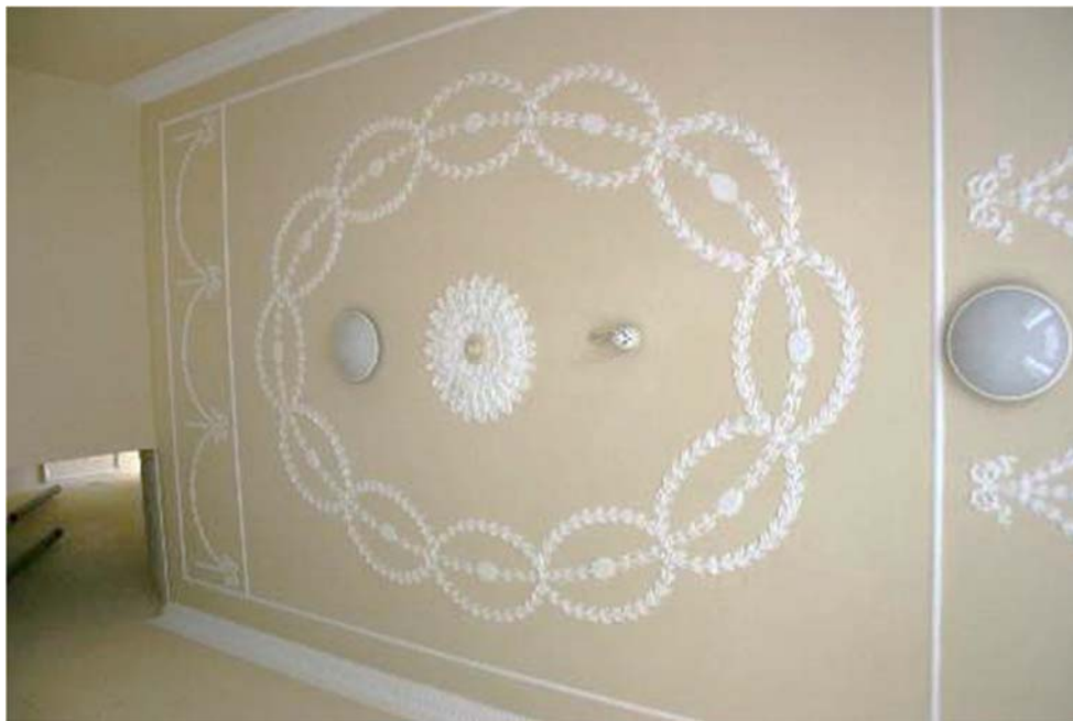
Plate 8: No 18 Entrance hallway, decorative ceiling
