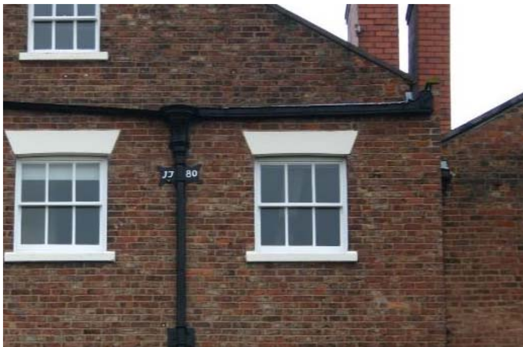
Plate 5: 1780 date plate at west facing elevation of 18 Nicholas Street
