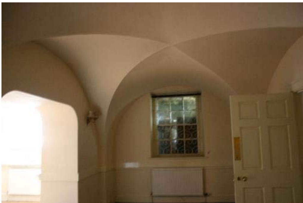
Plate 7: Cross vaulted ceiling in basement floor of No 18
