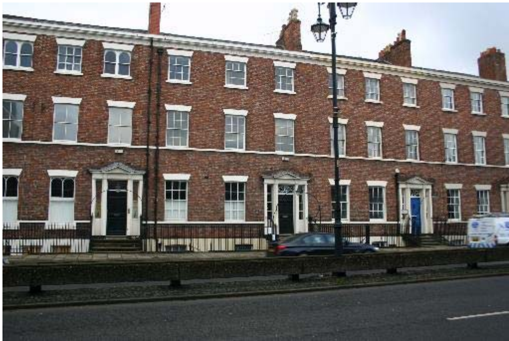
Plate 2: View of the east facing front elevation of 16-20 Nicholas Street
