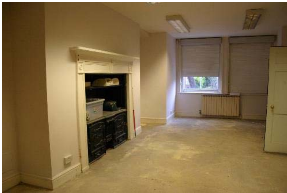
Plate 13: No 20 south-west room on Basement Floor
