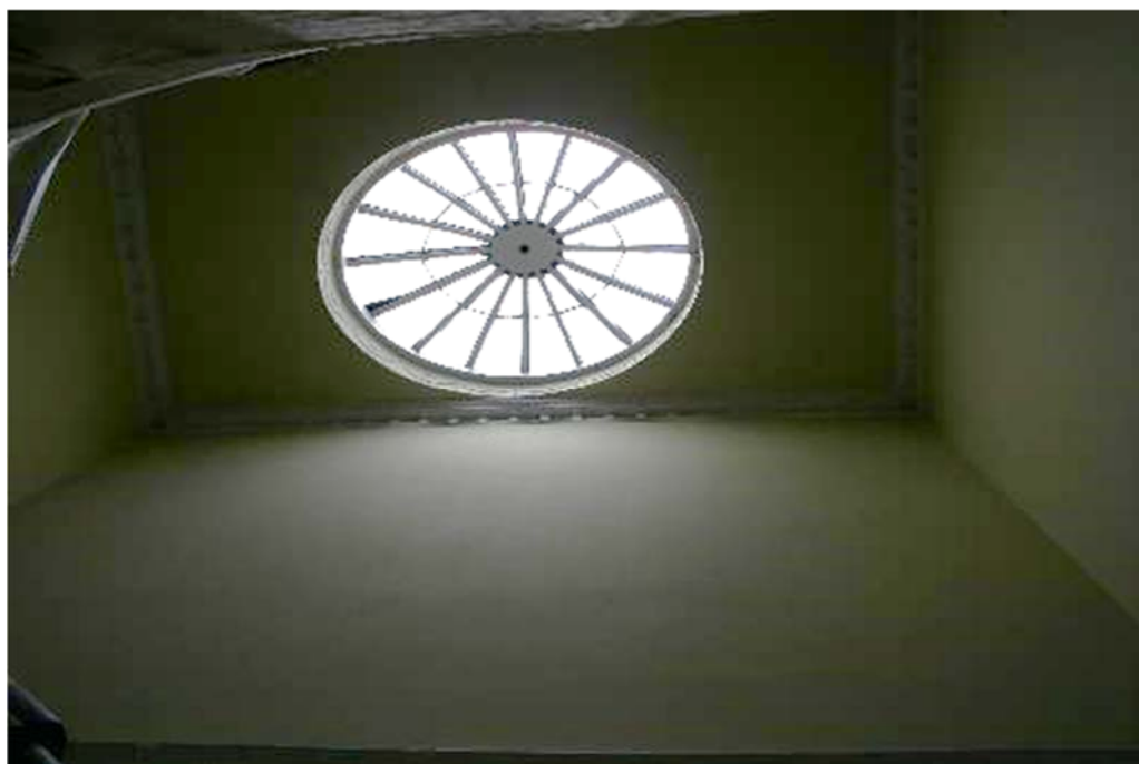
Plate 11: No 18, view of oval skylight at main staircase
