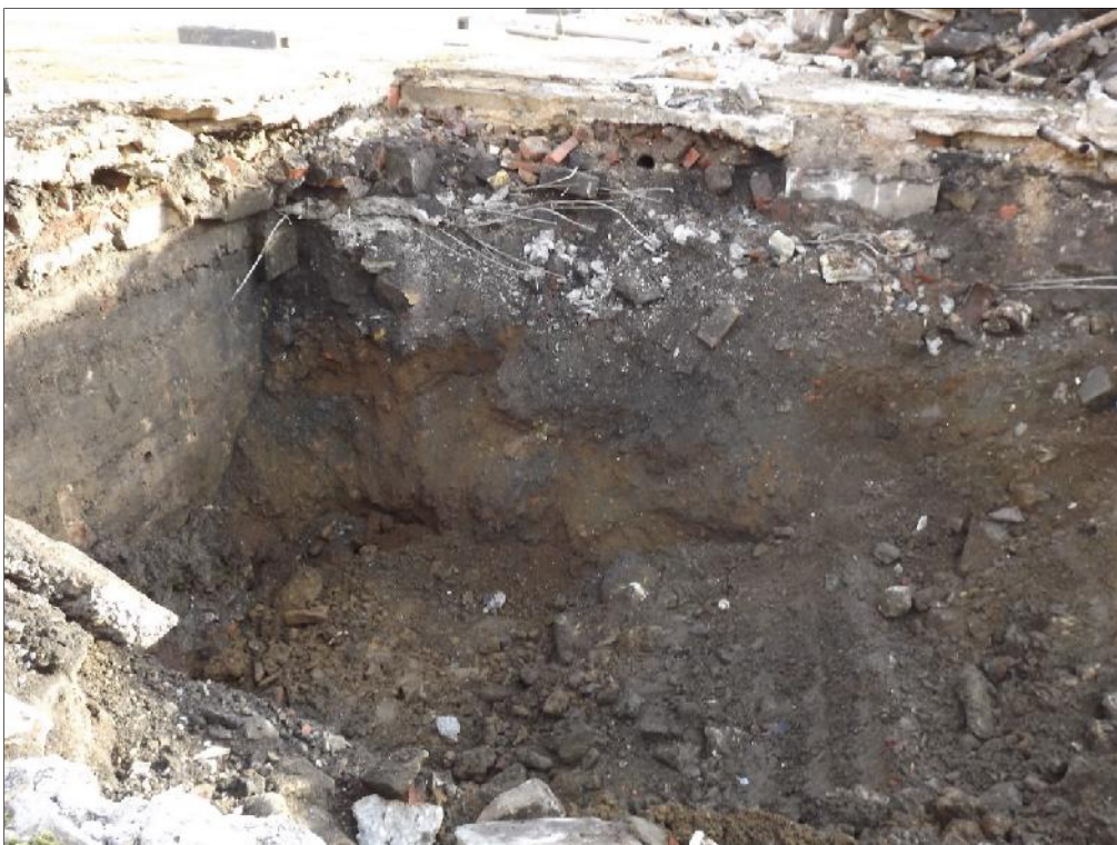
Plate 4: fully excavated trial pit 101, facing south.
