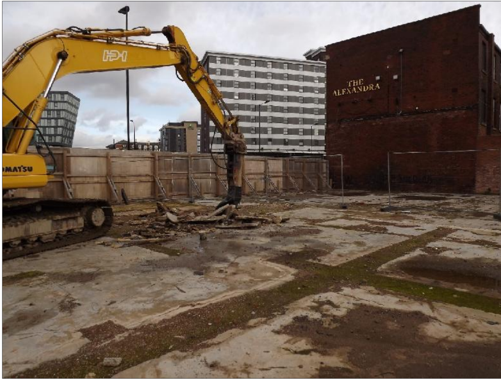
Plate 1: Removal of Concrete surface (100), facing north-east.
