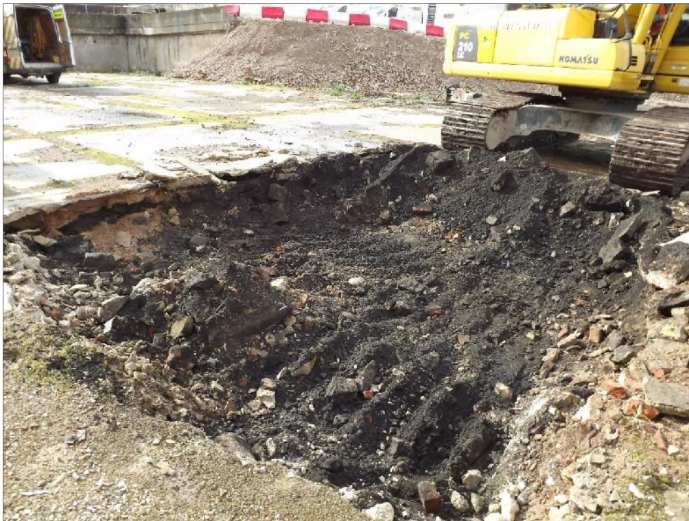
Plate 2: Showing 20 th century demolition refuse (103), facing south-east.
