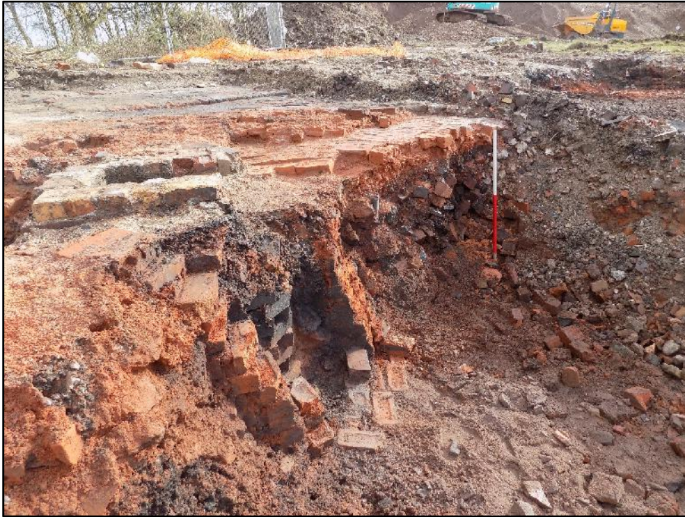
Plate 4: Oblique shot of the truncated west-southwest-facing elevation of kiln base {105} and central downdraught flue {117}, looking SE, 1x1m scale
