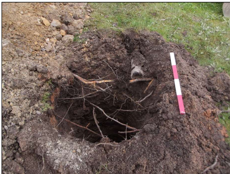
Plate 1: Hole excavated for new electric pole; looking east
