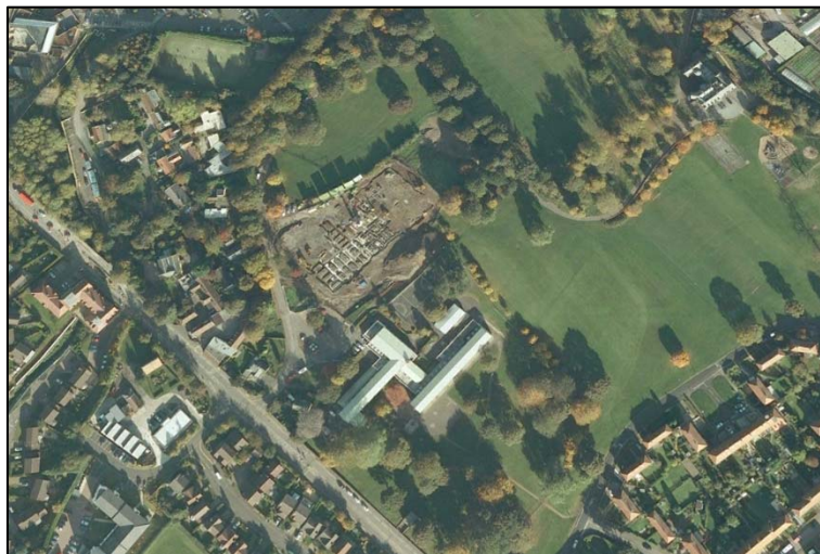
Plate 2: Google Earth Imagery showing demolition of school/ construction of care home, 1 st January 2009
