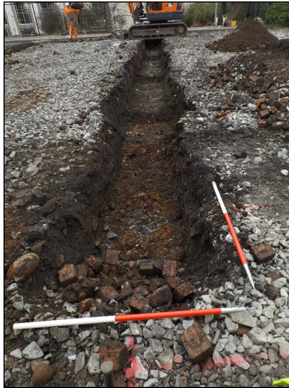
Plate 5: Showing the north-western foundation trench for the new building, facing south-west
