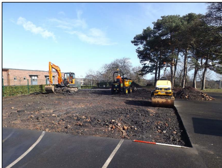
Plate 4: Showing initial ground reduction of building's footprint, facing north-east
