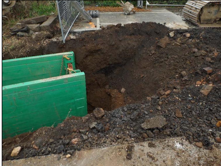
Plate 7: Showing excavations for the new personnel access chamber, facing north-west
