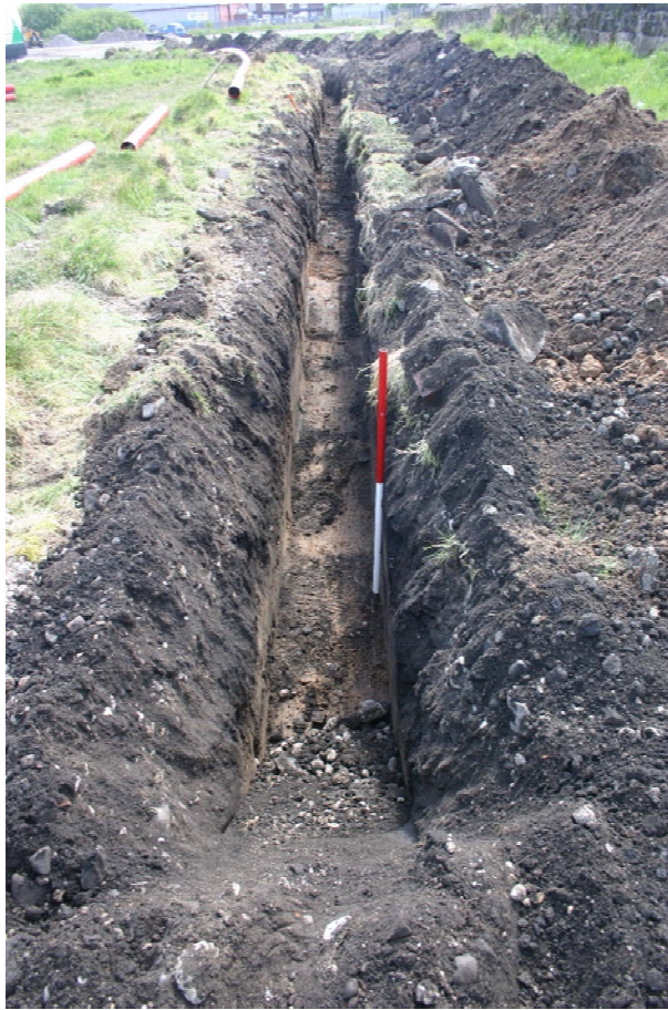
Plate 7: view of the trench, begin of sand deposit
