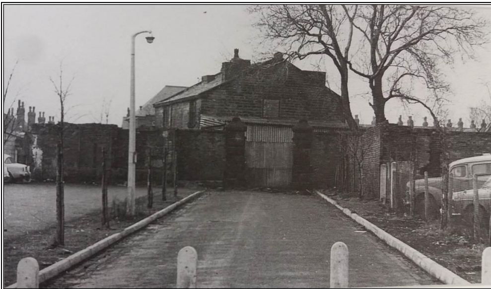
Plate 2; 1960s view looking south-west showing the gates to Primrose Cottage, with Primrose Cottage beyond, and Moor Street devoid of housing (Source: Smith 2002).
