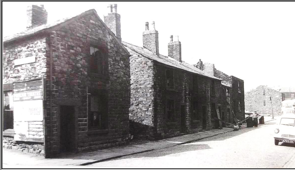
Plate 1; Fleet Street, showing house numbers 1, 7, 9, 11 and 13 (view looking north from Gillibrand Walks), in the process of demolition in 1962 (Source: Smith 2002).
