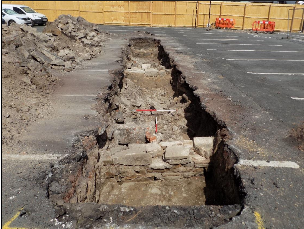
Plate 3; Trench 1, looking north-east, 2x1m scales.
