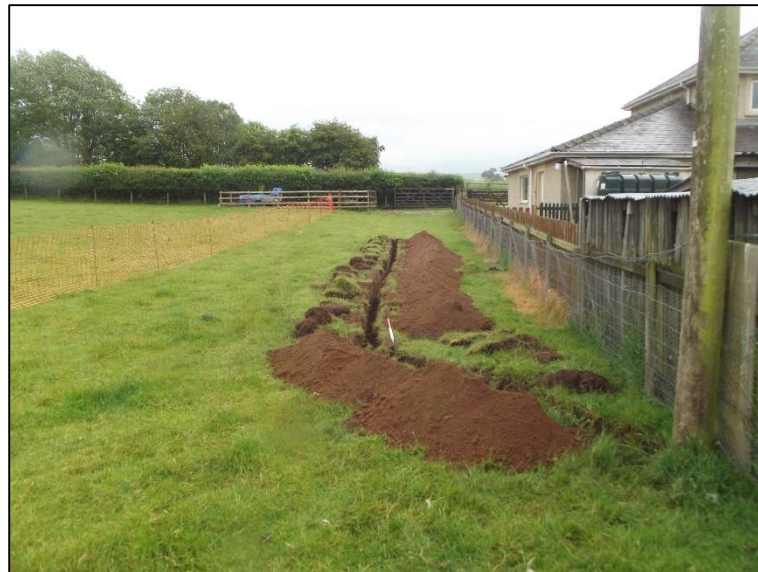
Plate 4: Cable trench, showing change in orientation, facing south-west
