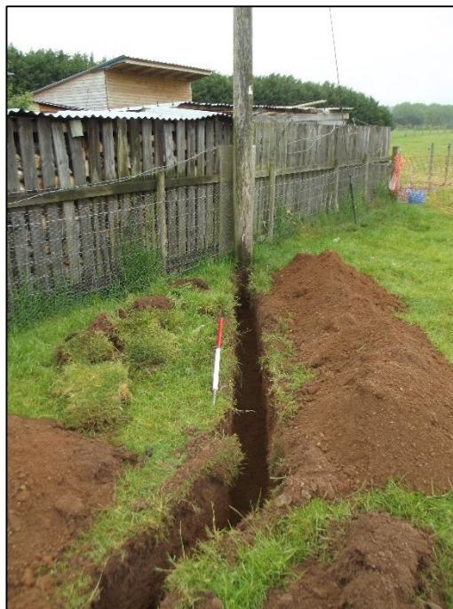
Plate 3: North-western extent of cable trench, facing north-west
