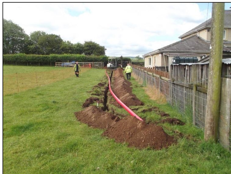
Plate 5: Cable trench once completed, facing south-west
