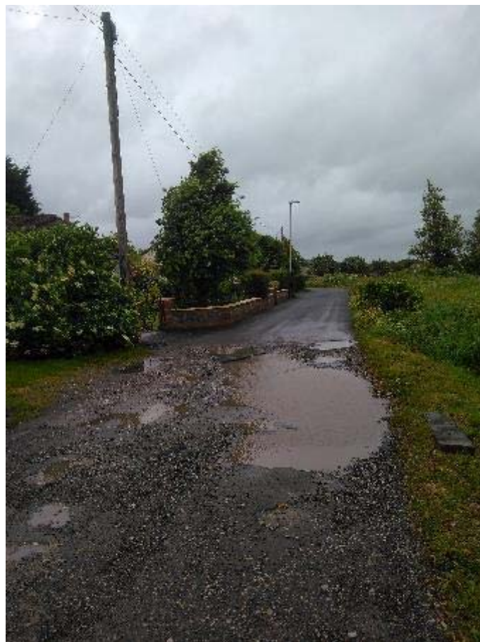
Plate 5: Nicholas Street towards site
