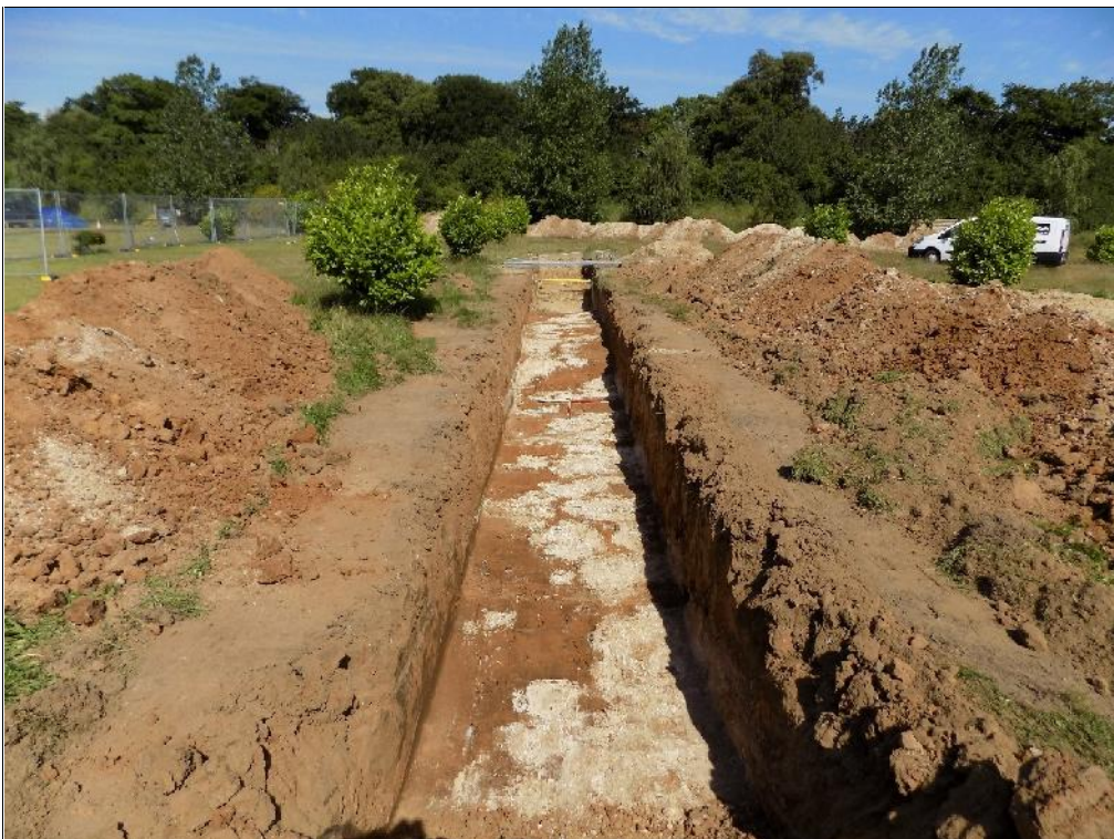
Plate 12: View of Trench 10 showing chalk substrate, looking northwest
