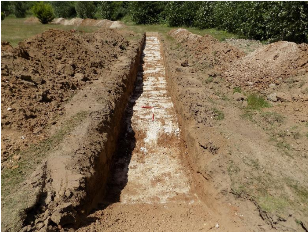
Plate 3: View of Trench 3 showing chalk substrate, looking northwest
