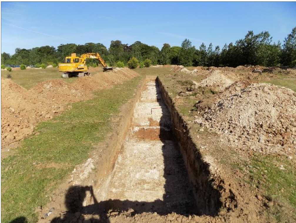
Plate 6: View of Trench 5, looking northwest
