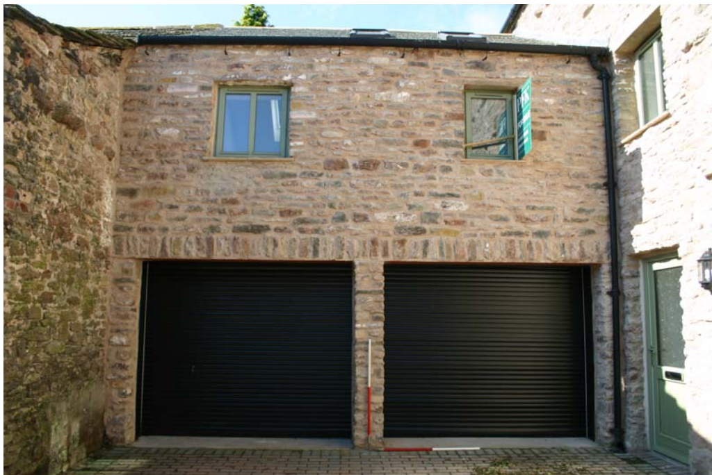
Plate 5: Partially rebuilt garage building
