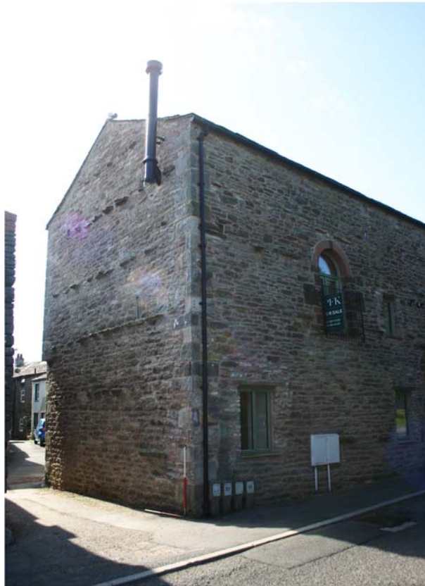
Plate 1: North facing elevation
