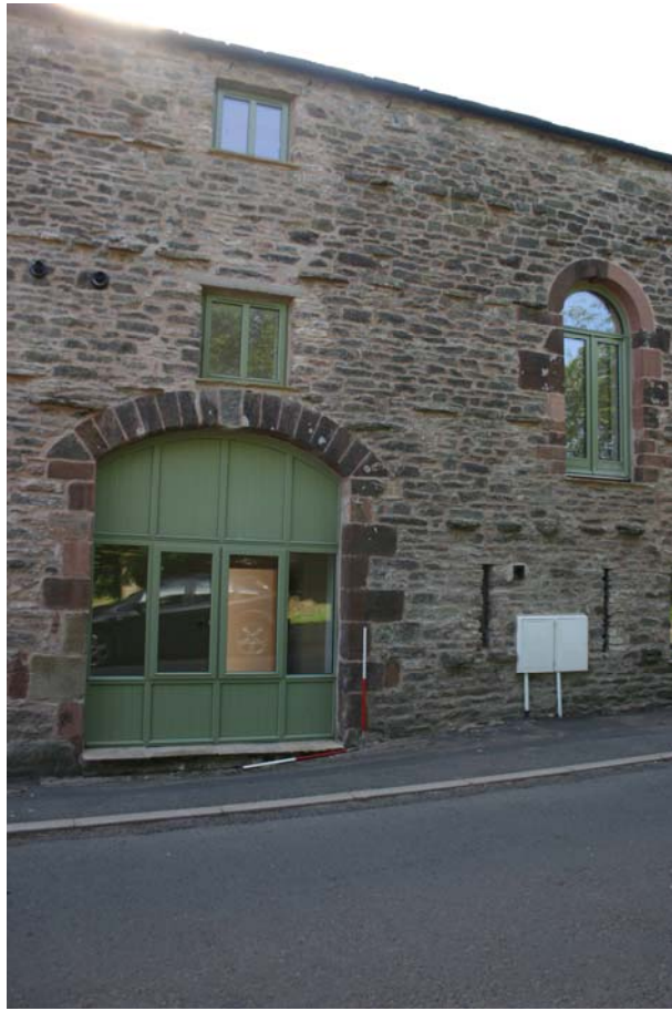
Plate 8: Detail west facing elevation, segmental arch and round arched opening
