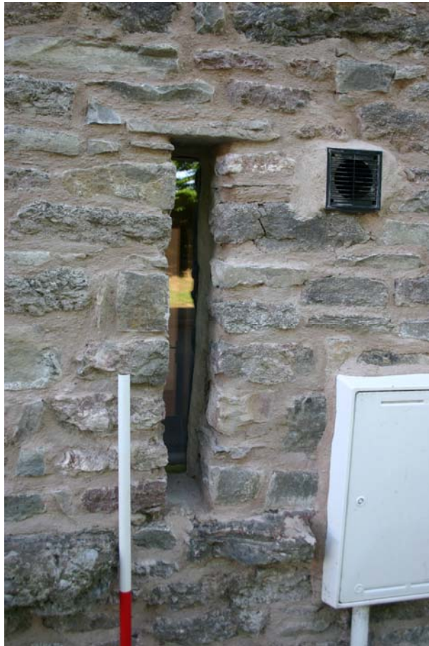
Plate 9: Detail, west facing elevation, narrow ventilation slit, modern glazed
