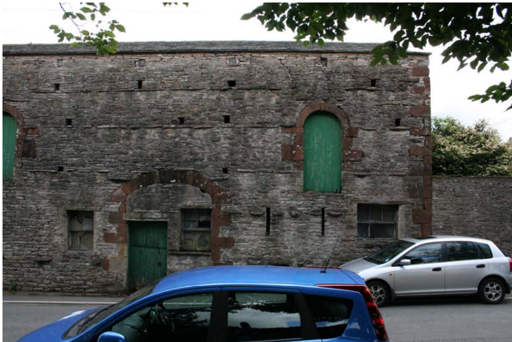
Plate 19: Detail south end of west facing elevation prior to development, by Graham K Norman Architect
