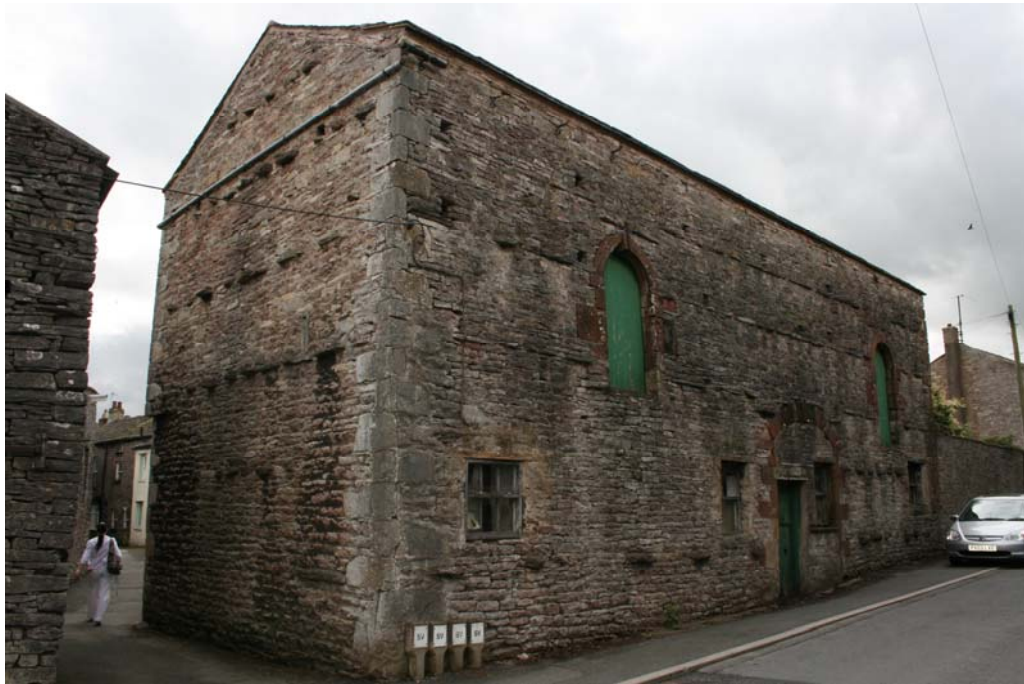
Plate 18: West facing elevation prior to development, by Graham K Norman Architect
