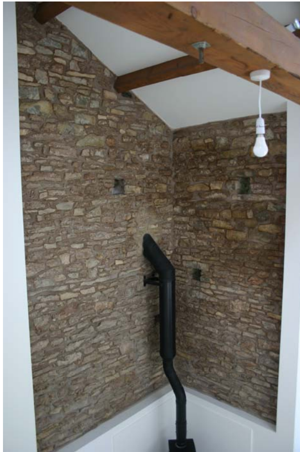
Plate 13: Interior southern building, exposed masonry at first floor living room
