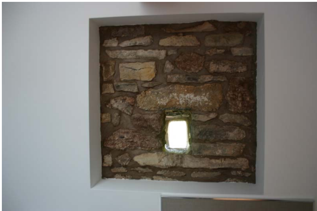
Plate 12: Interior northern building, exposed masonry and glazed opening
