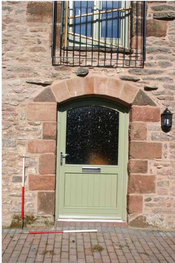
Plate 3: Detail, east elevation segmental arched doorway
