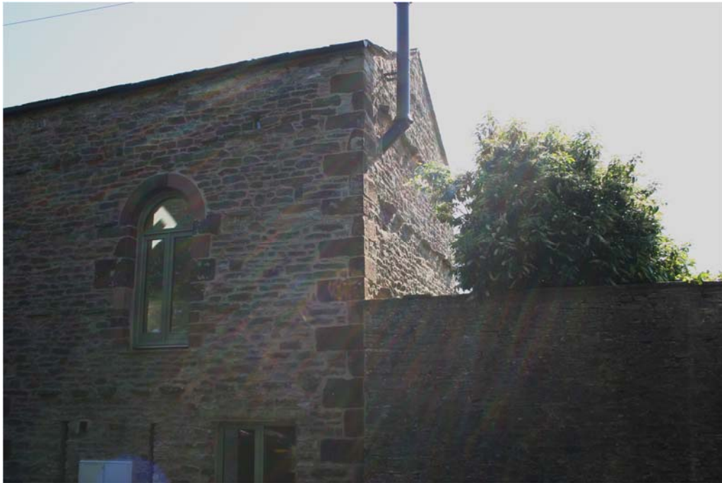
Plate 6: South facing elevation
