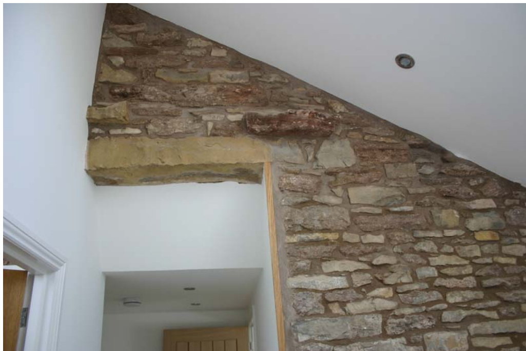
Plate 14: Interior southern building, exposed masonry with sandstone lintel
