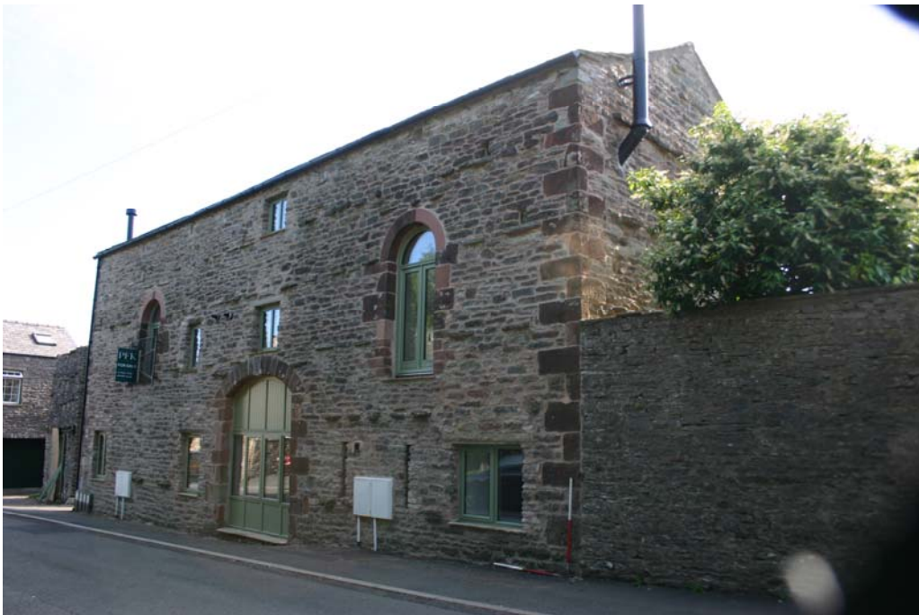
Plate 7: West facing elevation
