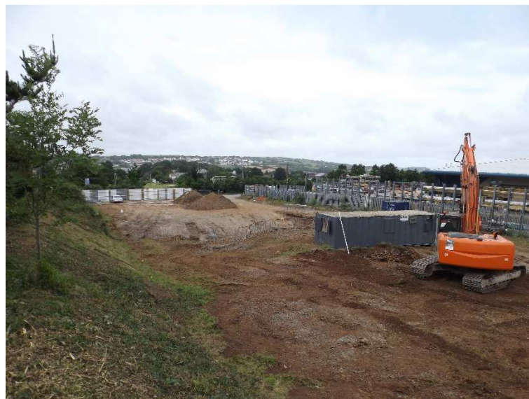
Plate 10: Completed ground reduction from north-east corner of site, facing west
