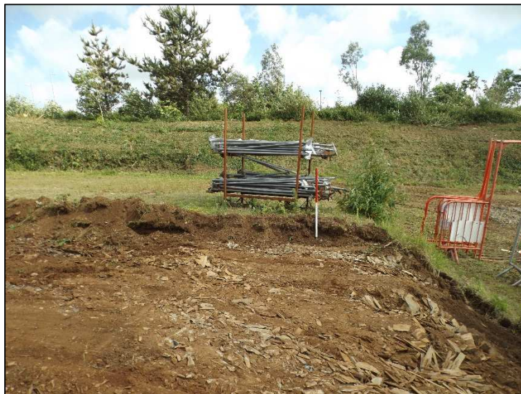
Plate 6: Revealing topsoil towards north-east corner of site, facing north-east
