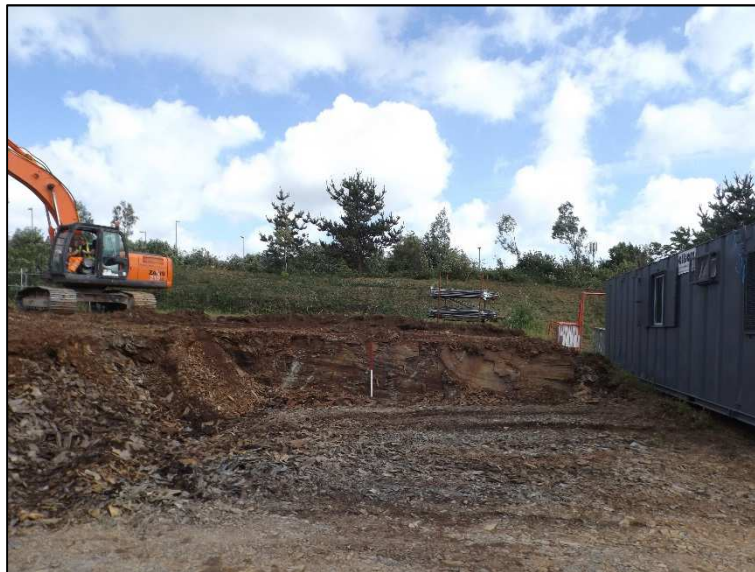
Plate 5: Ground reduction towards north-eastern part of site, facing north-east
