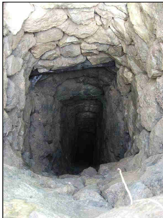
Plate 16; Feature 15 (Shaft 7) showing wooden beam supporting ginging - looking north
