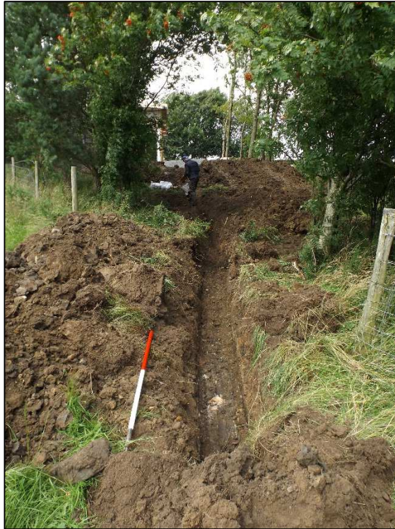
Plate 5: Southern extent of service trench, facing north
