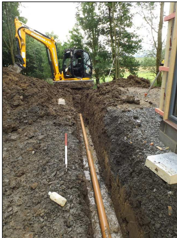
Plate 4: Service trench east of east bedroom module cluster, facing south
