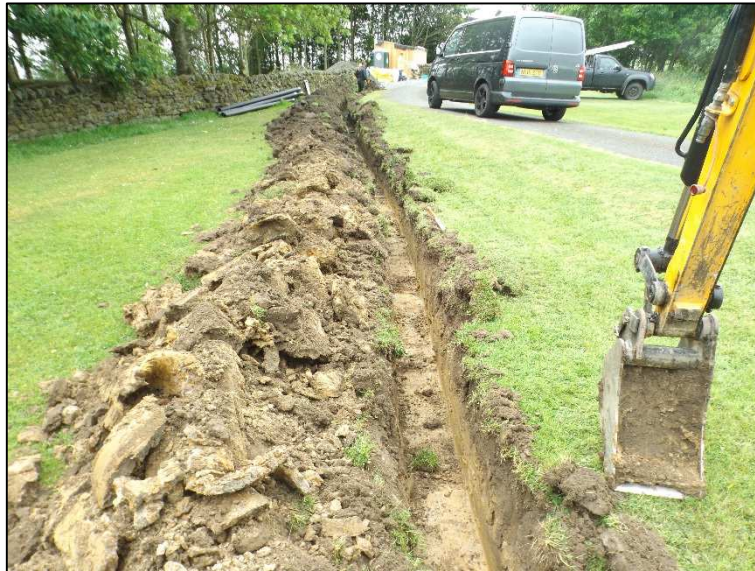
Plate 2: Cable trench, facing west
