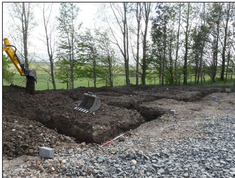
Plate 1: Foundation trenches for eastern bedroom module cluster, facing south-west
