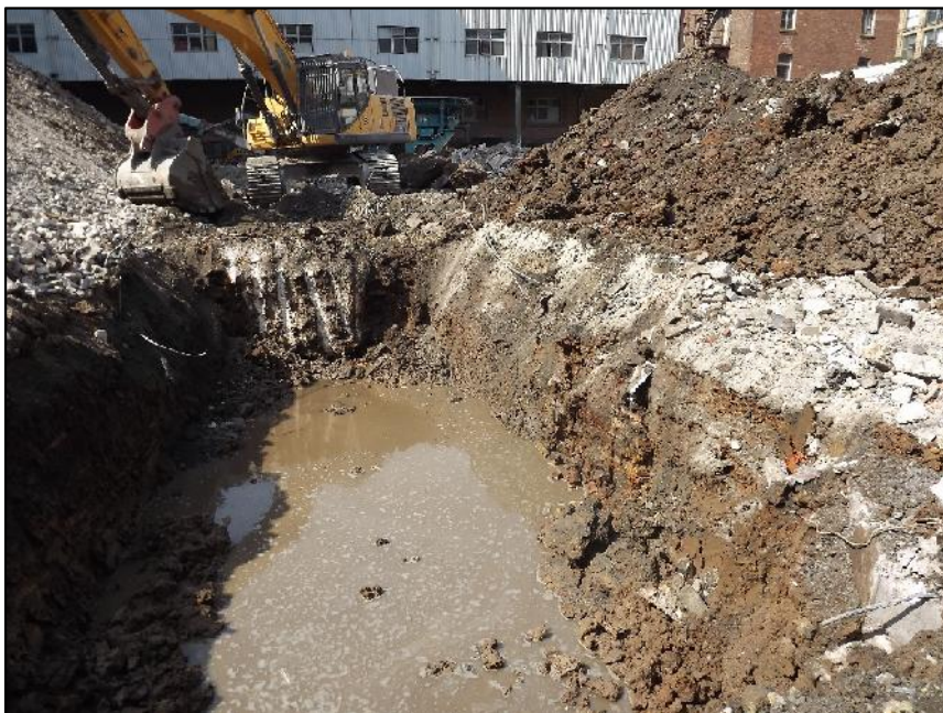
Plate 10: View looking west showing a section of brick wall in the south facing section (right of photograph), Block C (June 2017)
