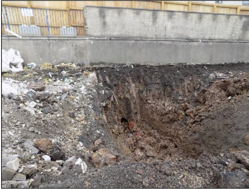
Plate 5: Section of brick culvert exposed during excavation of Block C (June 2017)
