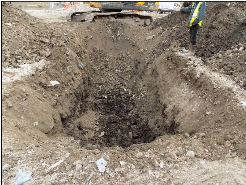
Plate 12: Detail of excavated test pit, Block F (August 2017)
