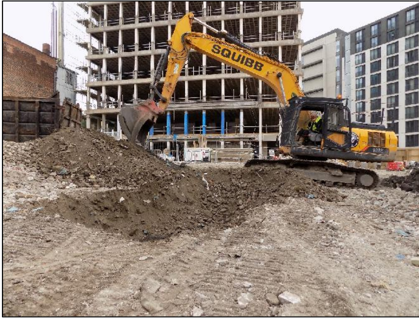
Plate 11: View looking north-east showing the groundworks at Block F (August 2017)
