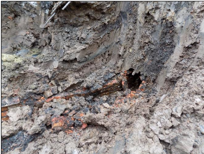
Plate 6: Detail of brick culvert exposed during excavation of Block C (June 2017)
