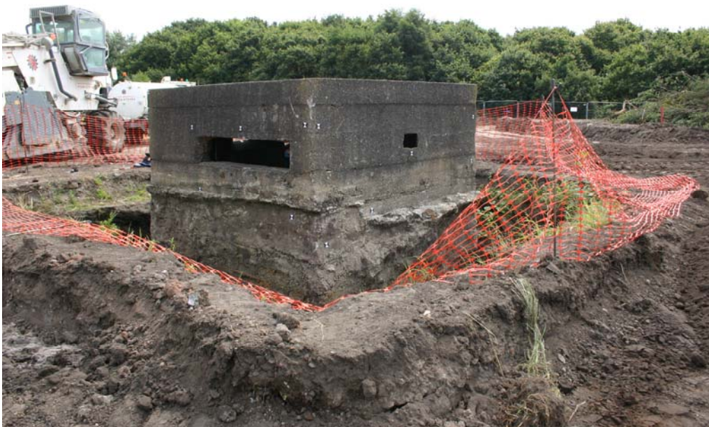
Plate 5: West facing corner
