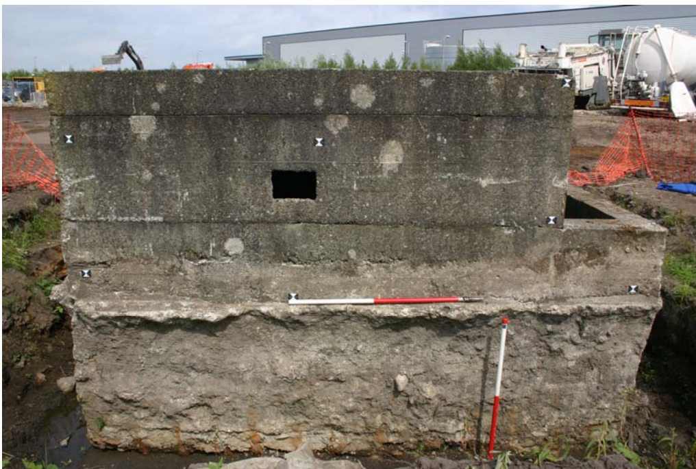
Plate 7: South-east facing elevation
