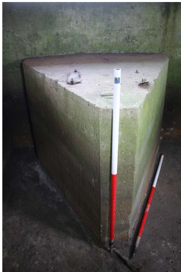
Plate 11: Interior, large, triangular concrete table to mount weapon on tripod
