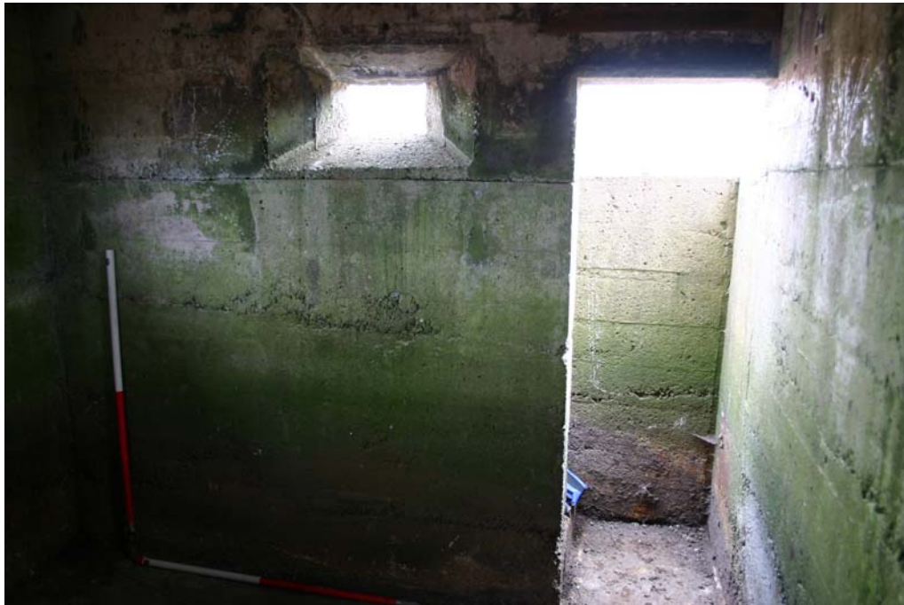
Plate 10: Interior, entranceway with small opening
