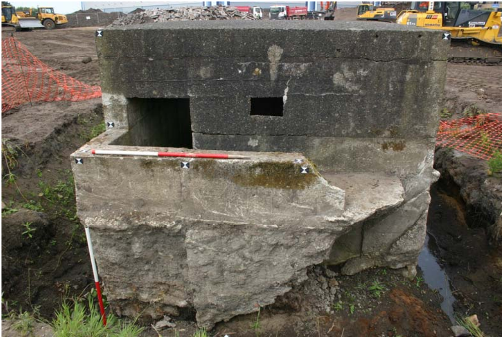
Plate 4: North-east facing elevation
