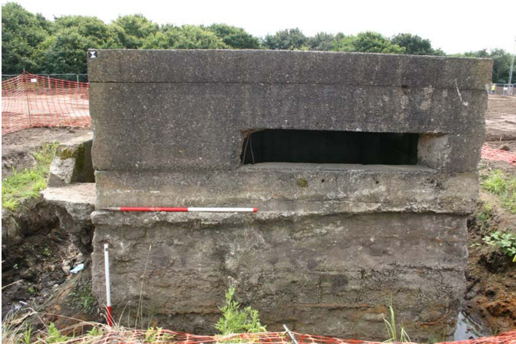
Plate 6: North-west facing elevation
