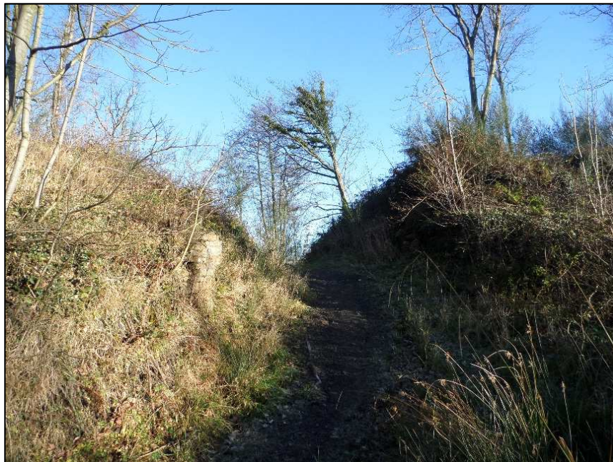
Plate 22: Bridge Abutments (A1.10, Asset 95) at site visit, facing north-east
