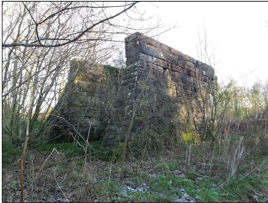
Plate 25: Remains of former buildings (A1.10, Asset 88) at site visit, facing north-west
