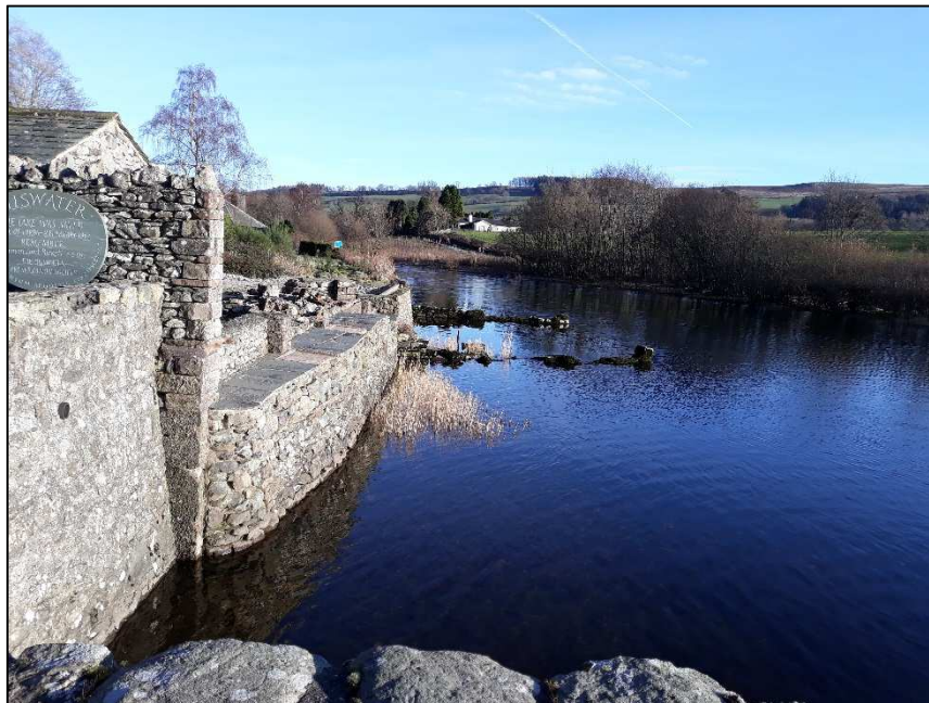
Plate 26: The remains of the jetties (A1.2, Asset 13)
