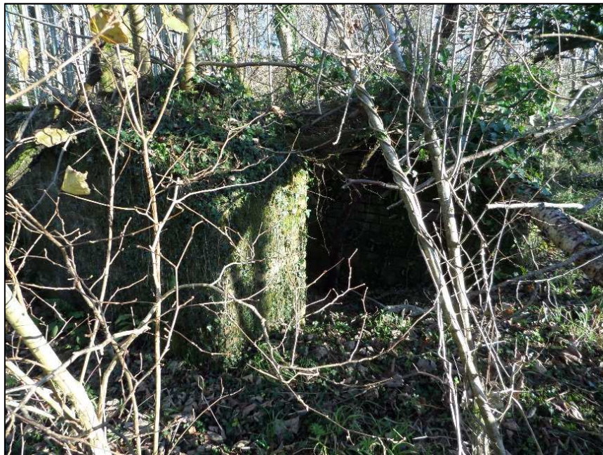
Plate 24: Shaft (A1.10, Asset 90) at site visit, facing north-east
