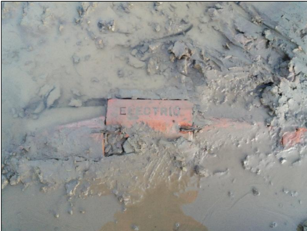
Plate 1; PHASE 1 - detail of electric cable, facing east with no scale
