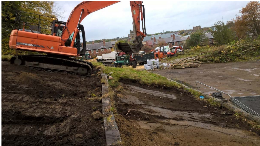
Plate 2: View of Area 2 during topsoil strip (looking west)
