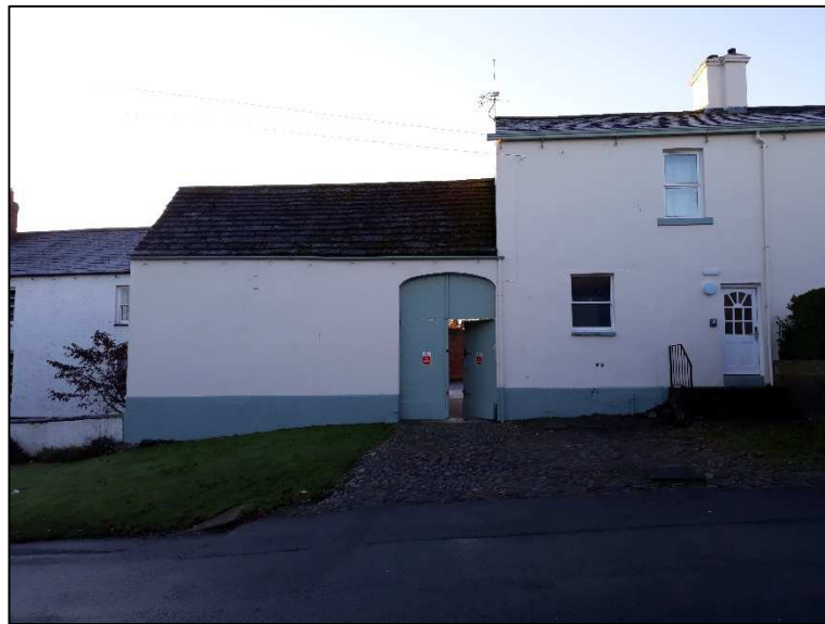
Plate 3: Access to evaluation site from Wood Street, facing south-east
