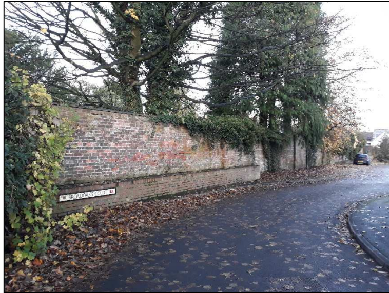
Plate 1: View of eastern boundary wall, facing north-west
