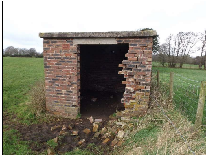
Plate 2: Brick-built hut at eastern boundary of field, facing north-west
