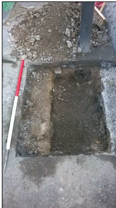
Plate 2: Trench 22 (looking east)
